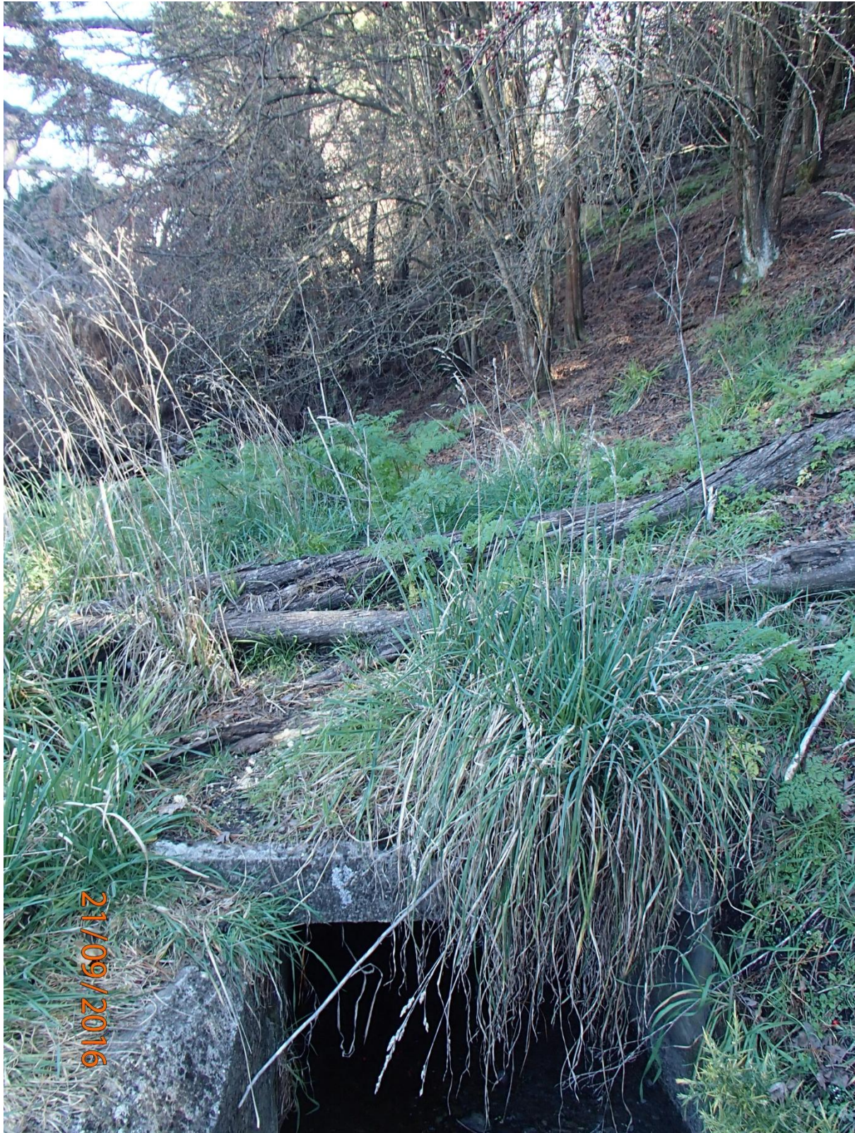
Photo 2: Lined and covered concrete tunnel over water race.
