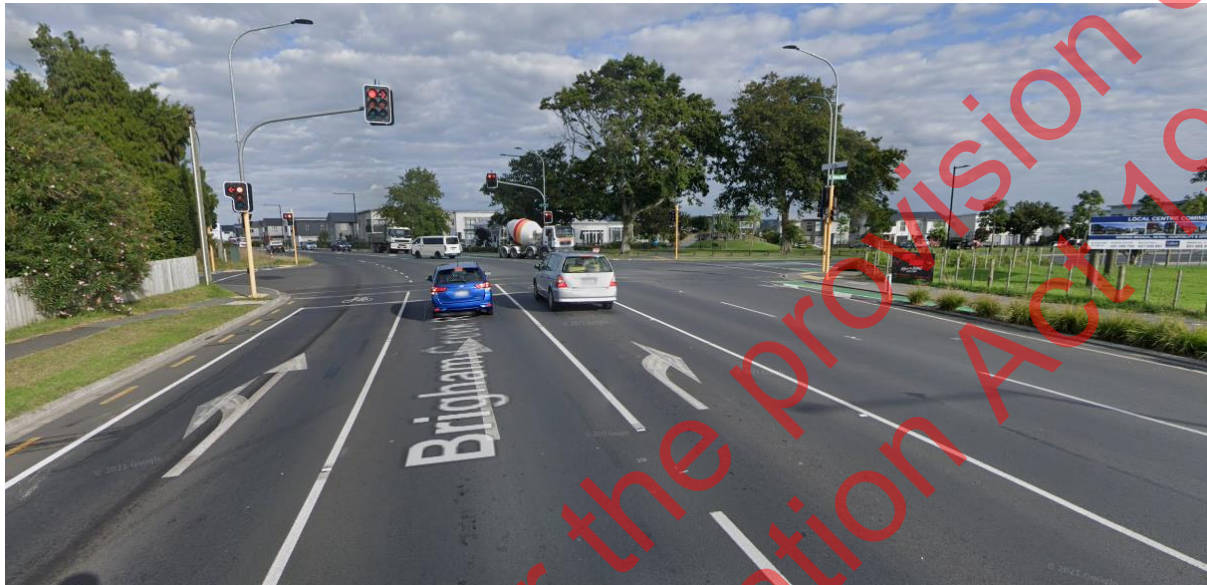
Figure 3: Completed upgrading of Brigham Creek Road within Whenuapai village (Source: Street View)
