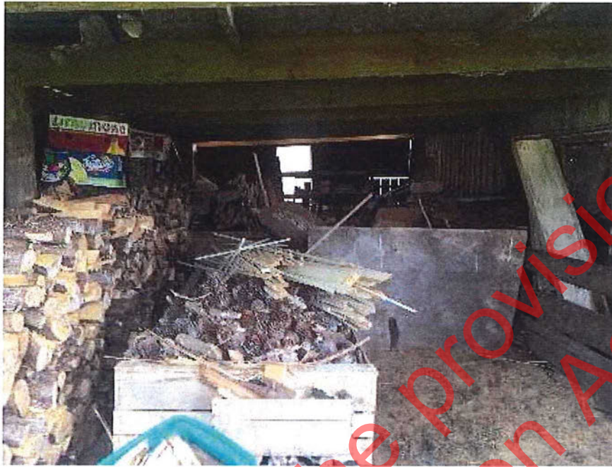
PLATE 7: INTERIOR OF BARN / TRACTOR SHED
