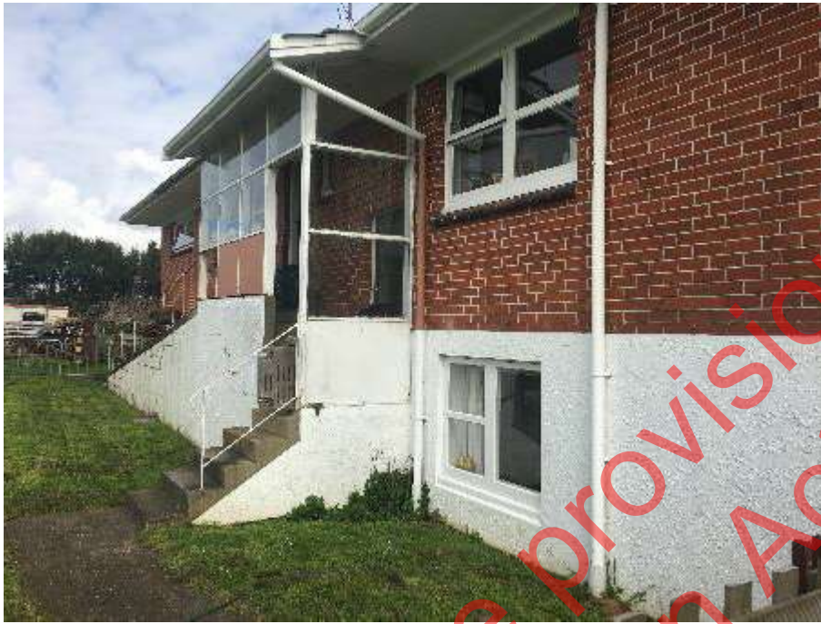
PLATE 3: EASTERN SIDE OF THE ORIGINAL DWELLING
