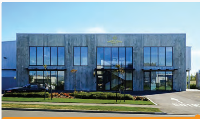
Stark Drive Original Foods, Christchurch
