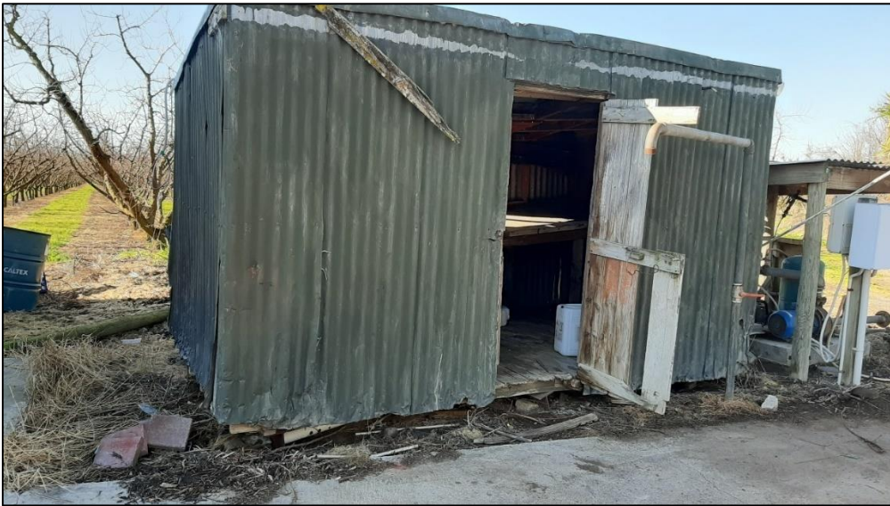
FIGURE 5. ABOVE GROUND FUEL TANK
