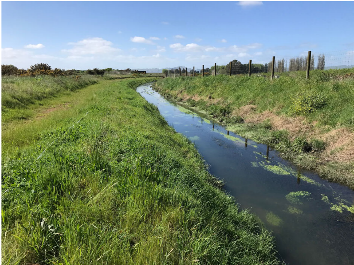
Figure 1. Typical character of the reach of the Wellwood Drain proposed for culverting.
