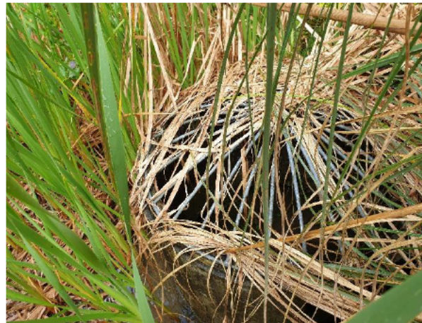
Photo 12. Scruffy dome installed within the constructed wetland.
