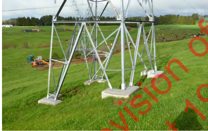
Left – Concrete encasement into wooden framework, Right – Completed works
