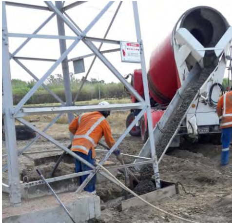
Left – Concrete encasement into wooden framework, Right – Completed works
