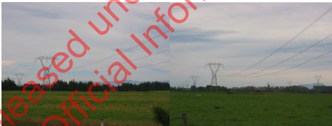
Left – Simplex conductor, Right – duplex conductor
