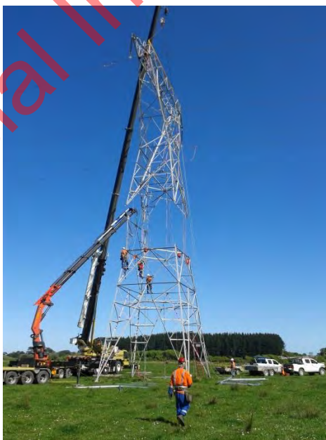
Example of a body extension in progress
