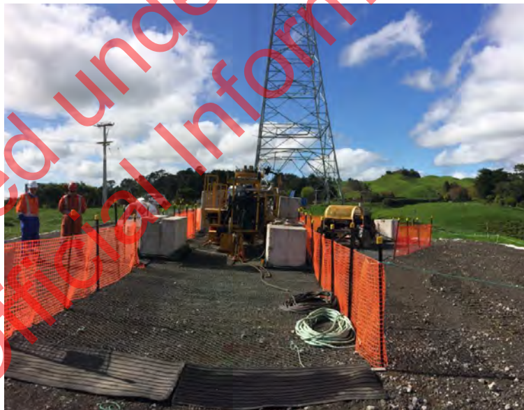
Wiring site with earth mat in the foreground
