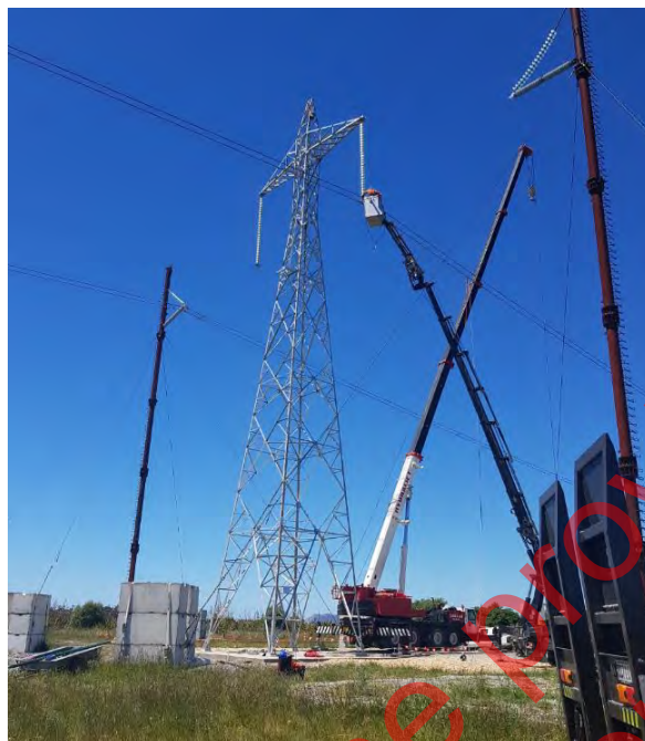
Insulator installation onto a newly constructed tower, using temporary structures.
