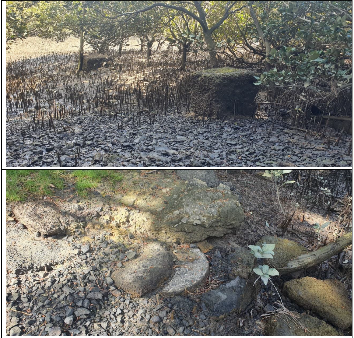
Figure 22. Photographs showing concrete piles on the northern side (top) and concrete structures on the south side of the boat ramp (bottom)
