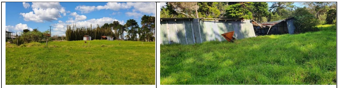
Figure 24. Photographs showing the bamboo fencing and dilapidated sheds separating the central and western portions of 101 Totara Road (left) and the collapsing corrugated iron shed containing various horticultural items (right)
