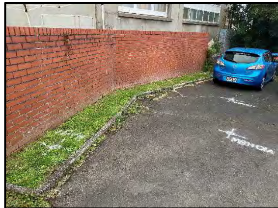
Photo 2: Eastern boundary toward the rear or the existing dwelling / café. Note: proximity of adjacent building to eastern property boundary, photo facing southeast.
