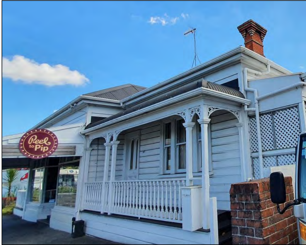
Figure 12 Northwest facing view of the eastern frontage of the historical villa building with a brick chimney visible and roll top verandah with fretwork.
