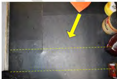
Fig. 26 Slight raise within the kitchen floor area aligns with the ceiling beam, indicating the edge and extent of original residential building.
