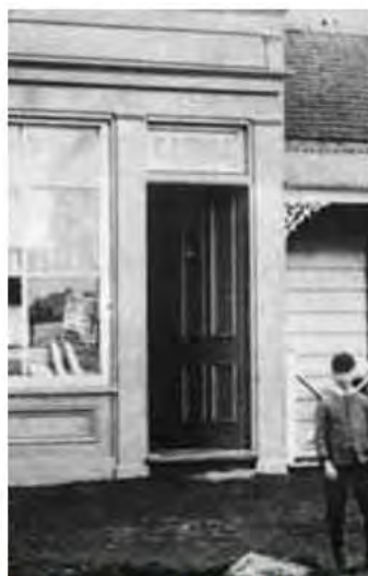
Fig. 30 The original door and transom window of the Momingside Store c1890s.
