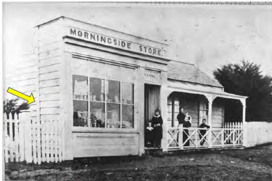
Fig. 9 Photograph showing the Morningside Store on the subject site circa 1880s. Note the misalignment of the weatherboards (indicated by the yellow arrow) suggests the shopfront window bay being a later addition to the original building (to the right). (Auckland Libraries Heritage Collections 255A-123)
