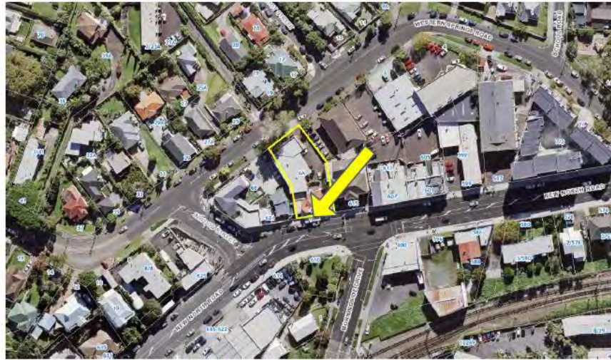
Fig. 2 Site aerial showing the site context, with the subject site (arrowed) at 617 New North Road, Kingsland. (Auckland Council GeoMaps GIS Viewer, 2022)
