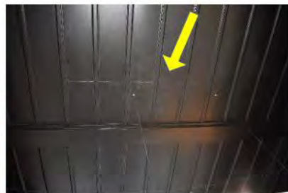
Fig. 27 A scarfing joint in ceiling suggests the presence of a chimney. Markings align with chimney shown in figure 18 and 20.
