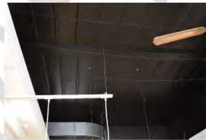
Fig. 25 Ceiling beam aligns with the extent of the original store / front of house area suggesting the extent of the residence.
