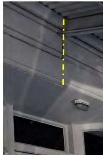
Fig. 29 A join within the weatherboards along the street front elevation indicates the extent of the original shopfront, aligning with the return wall within the café in figure 28.
