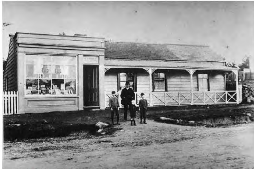
Fig. 6 Photograph showing the Morningside Store on the subject site circa 1880-1890s. The extent of the later addition to the right is distinguishable due to the colour variation on the shingle roof and the butt joins to the weatherboard. (Auckland Libraries Heritage Collections Map 4497-7)
