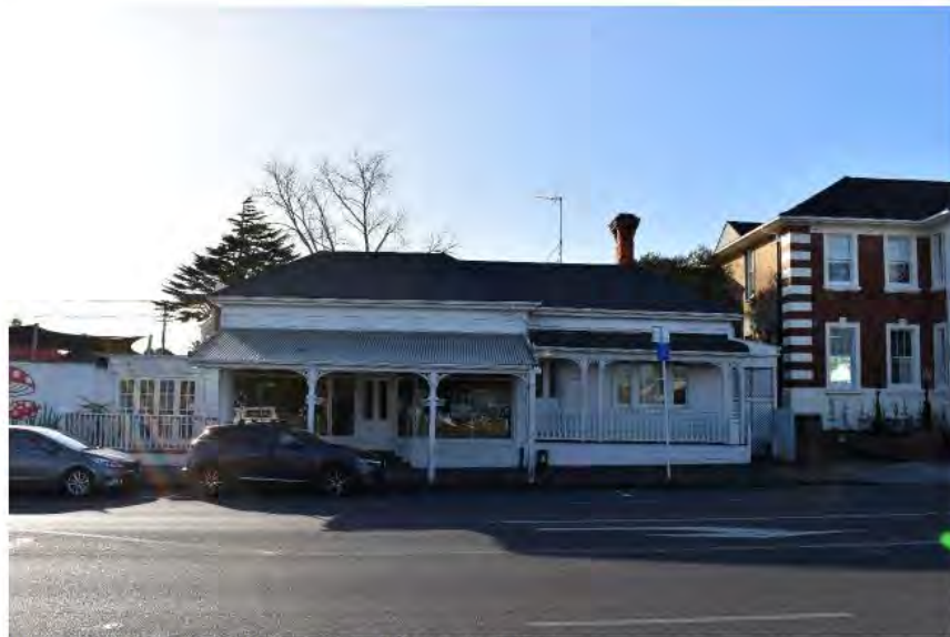
Fig. 3 Looking north towards the subject site at 617 New North Road.
