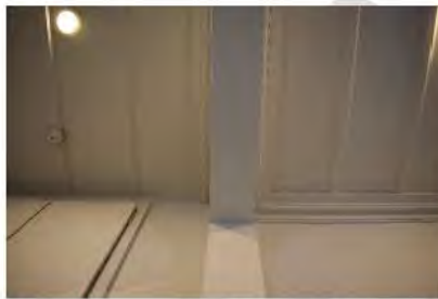
Fig. 24 Slight variation noted in the ceiling battens between the original c1880s building and the c1890s addition.
