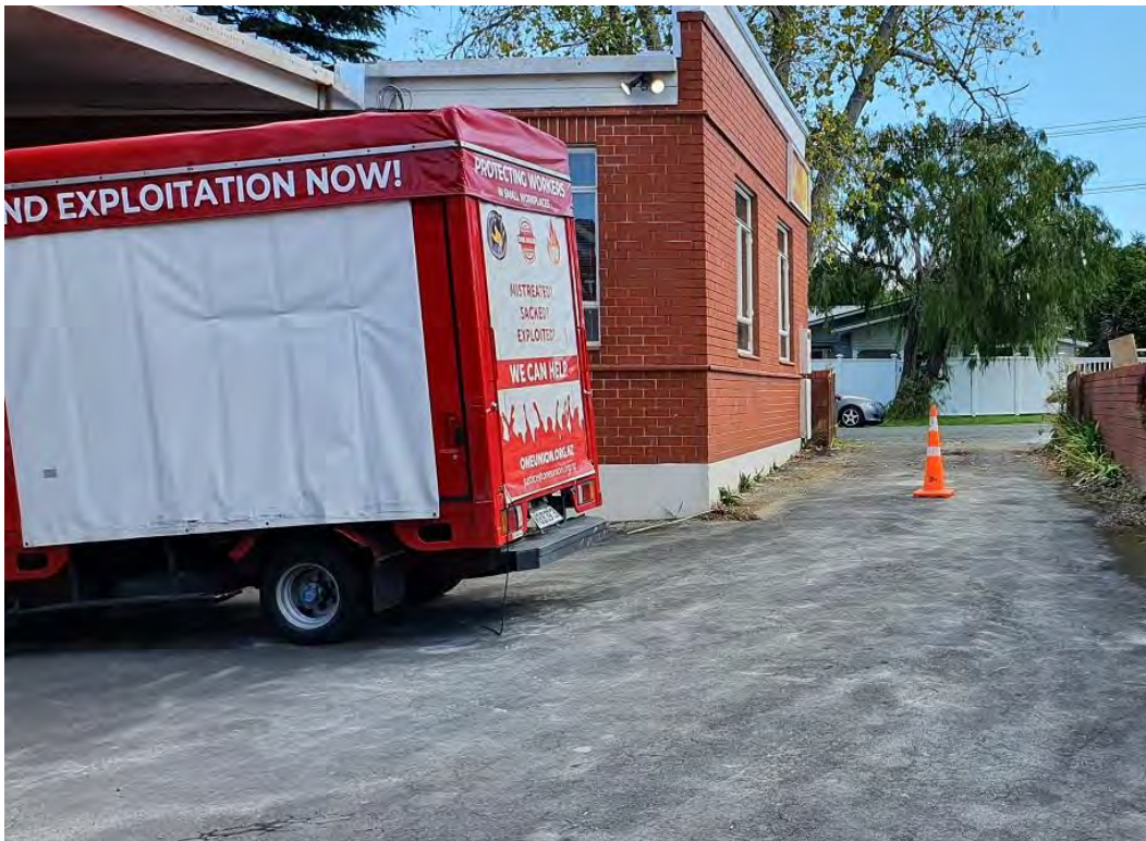
Figure 13 Looking north along the driveway and the eastern side of the later 20 th century brick built offices currently occupied by the Unite Union.
