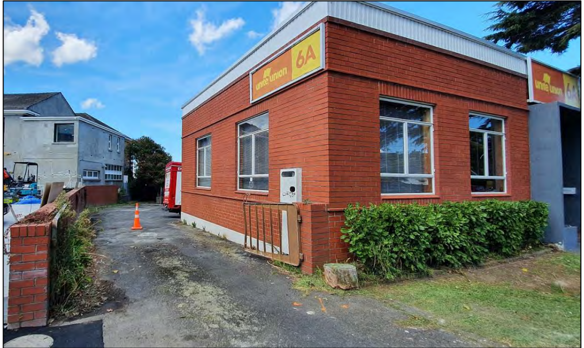
Figure 14 Looking southeast at the entrance to the office building and driveway fronting onto Western Springs Road.
