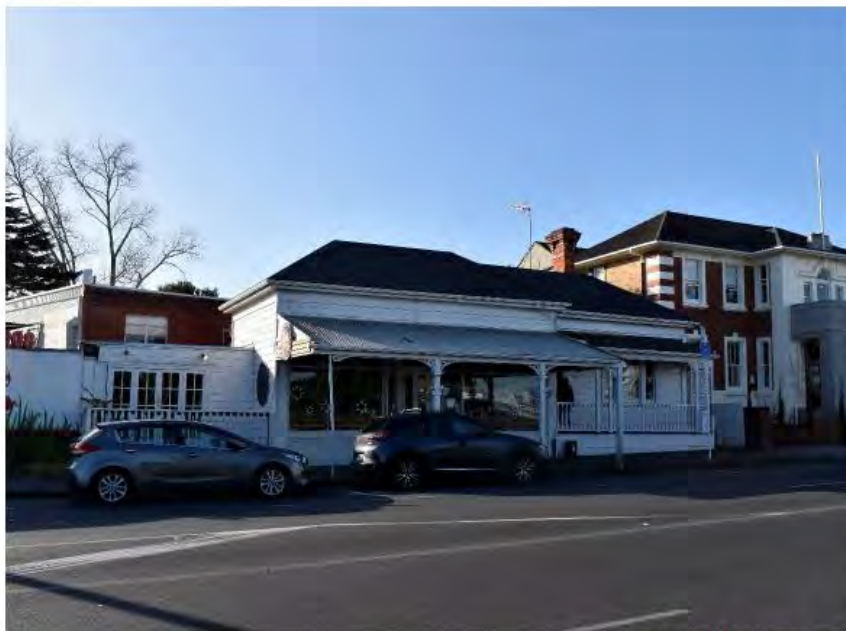
fig. 1 617 New North Road. (archifact – architecture & conservation ltd, 2022)
