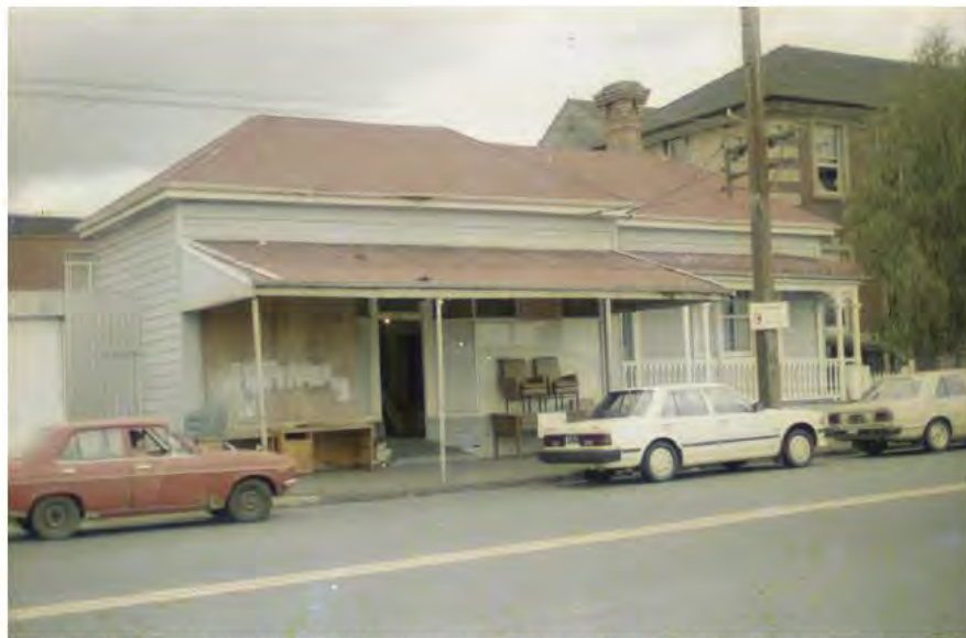
Fig. 7 The building at 617 New North Road has been subject to various additions and alterations between the earliest known photograph taken in c1880s and the photograph above taken in 1985. Note the extension to the shopfront window, the addition of a chimney, the change of the roof form, and alteration of the building's fenestration. (Auckland Libraries Heritage Collections Map 4497-7)
