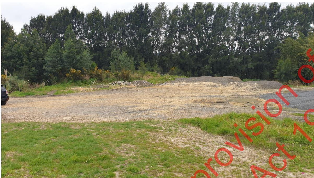
Figure 16. View looking north over earth worked area at southern end of block
