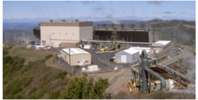
Figure 2. One of 22 dry steam plants at The Geysers in California.
