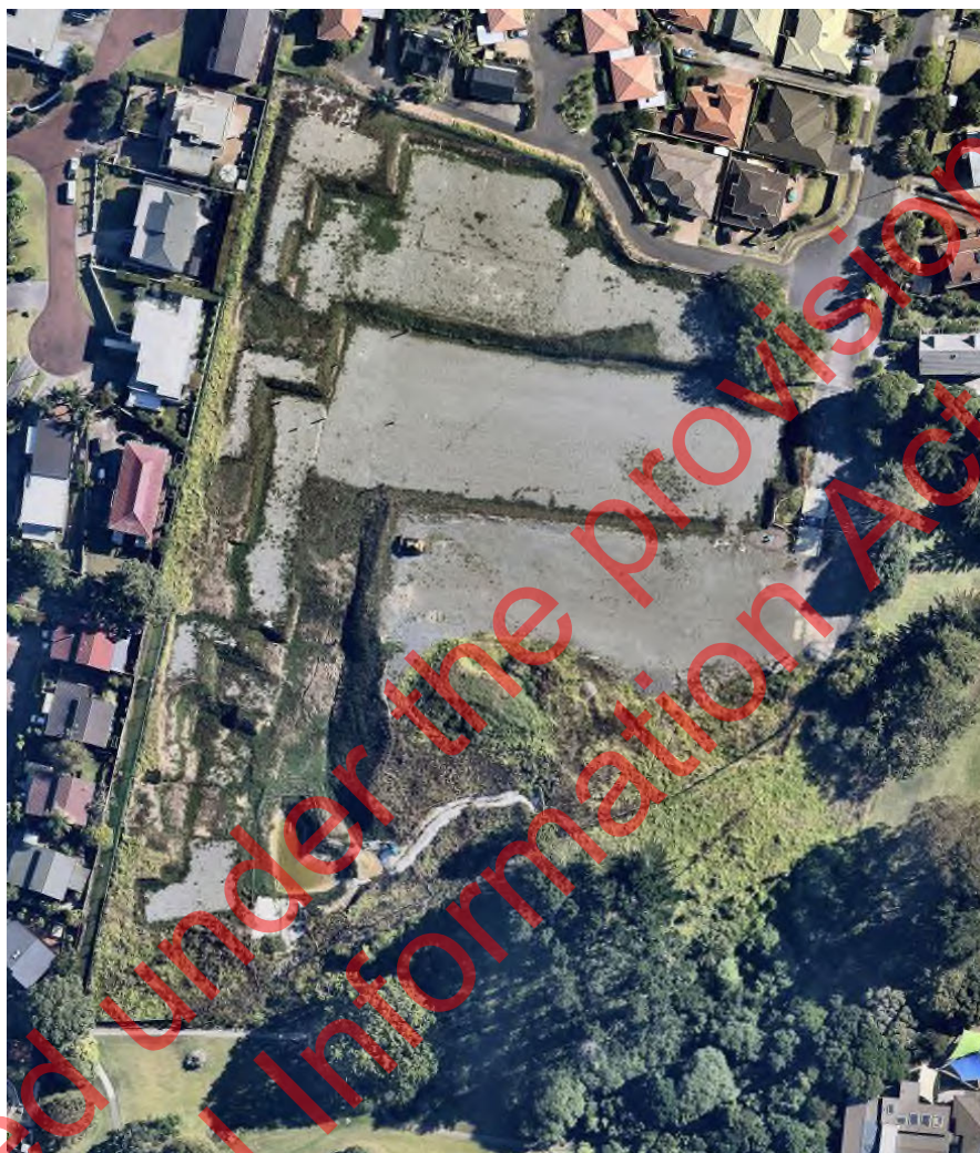
Figure 4: Stage One Bulk Earthworks
