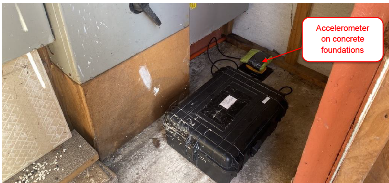
Figure 16 - Accelerometer on concrete foundations at Eastern end of existing building
