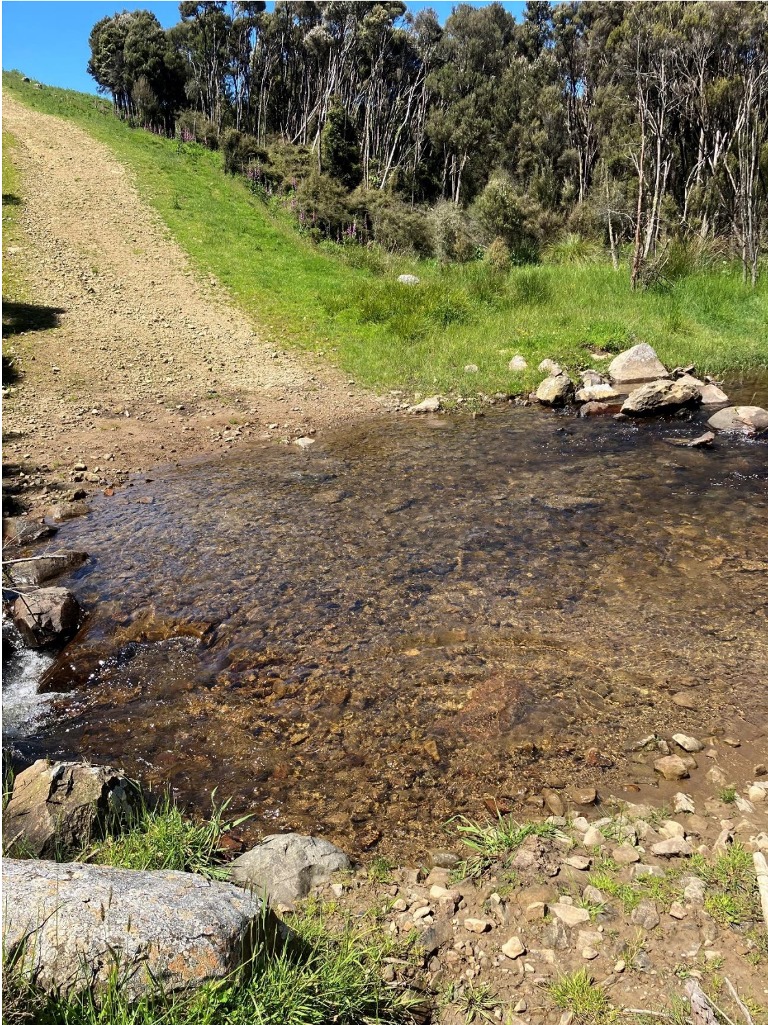
Plate A2.1: Ford crossing at Site 1, large gravel size and sufficient water depth ensures that fish passage is unlikely to be an issue during normal flows.
