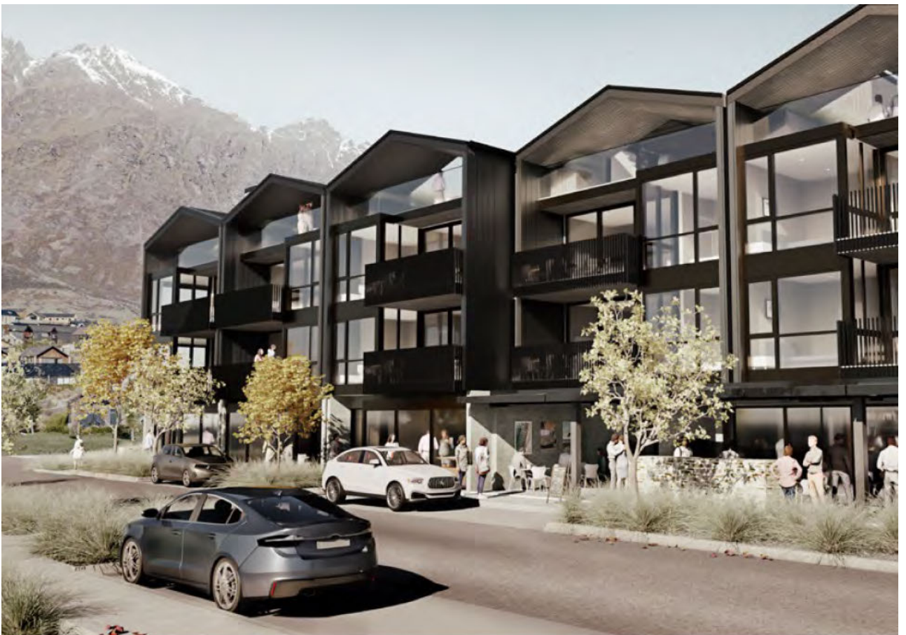
LOT 13 QUARTERS BUILDING – Production May 2023, installation from June 2023. Multistorey apartment building with CLT floors and HENZ walls and roof.
