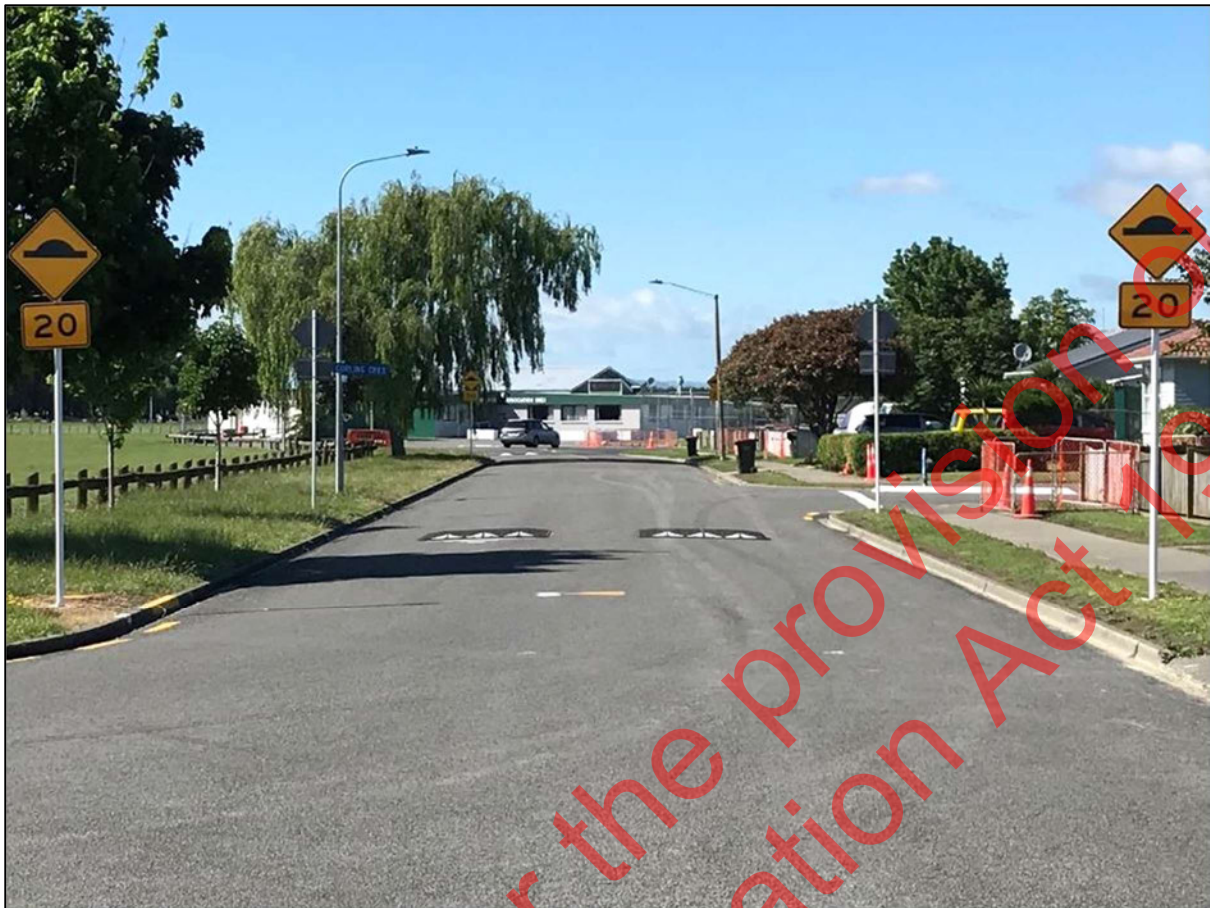
Figure 8 – Dinwiddie Avenue Southbound Photo (speed cushion and raised table traffic calming)
