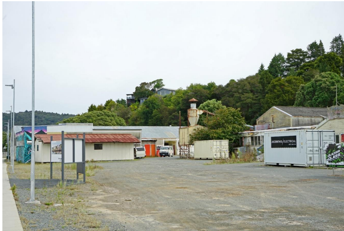
Photograph 2: Typical character of run-down buildings and yards on the site.
