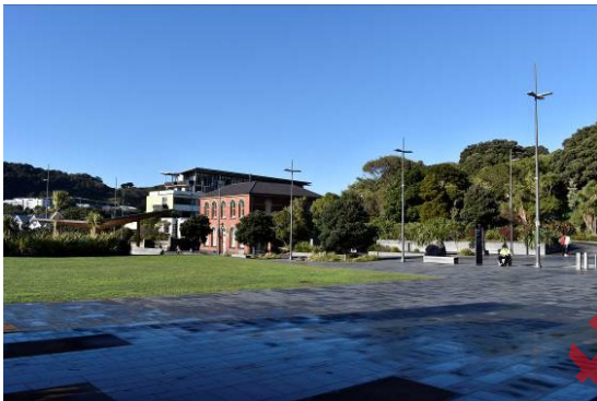
Fig. 25 Looking southeast towards the southeastern corner of the National War Memorial Park bookended by the former Mount Cook Police Station building, with the subject site beyond.
