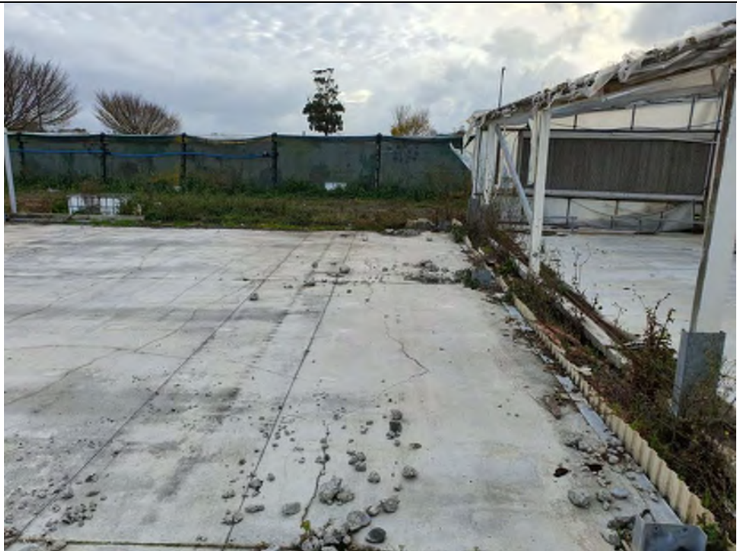
PLATE 6: RESIDUAL CONCRETE FOUNDATIONS WITH FIBREGLASS PRESENT ON EDGES.
