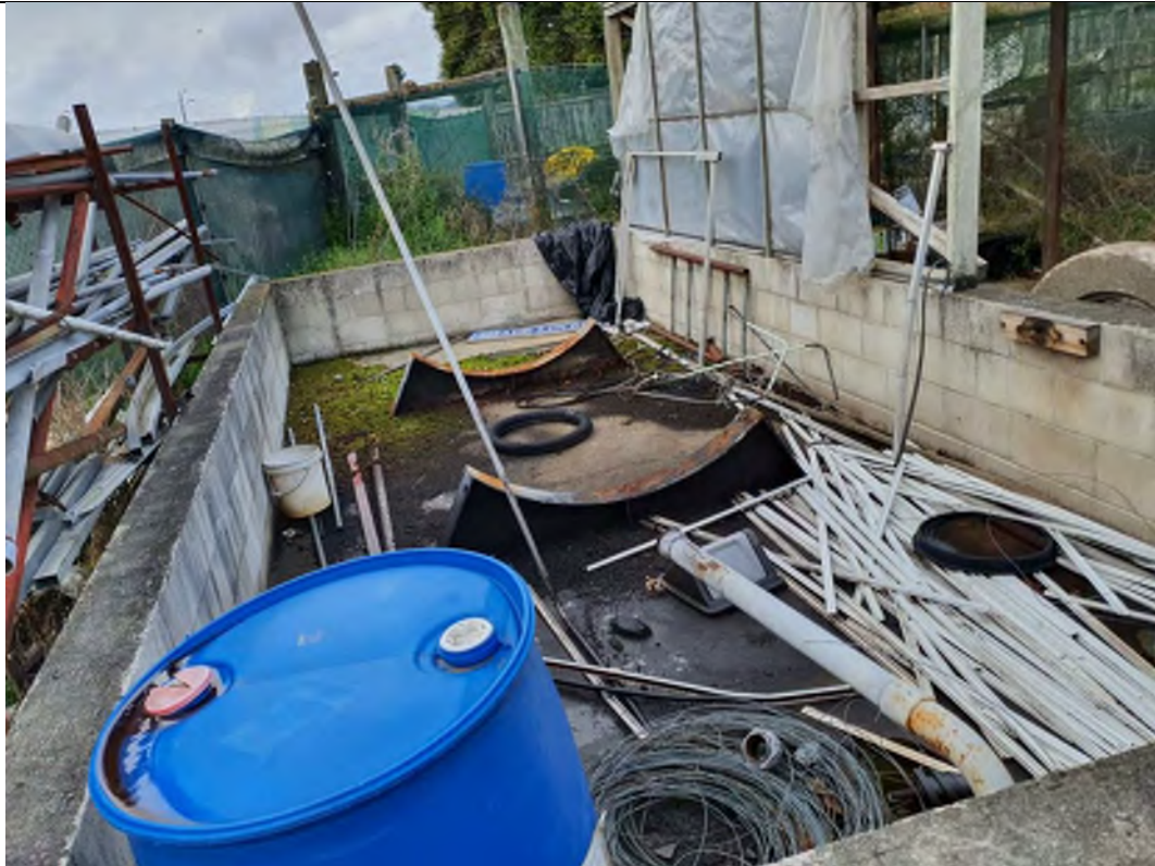
PLATE 3: FORMER DIESEL TANK BUND WITH STAINING EVIDENT IN FOREGROUND.
