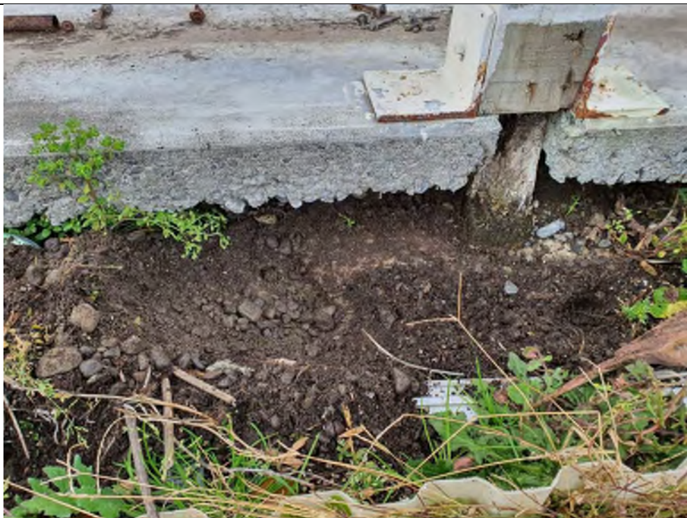
PLATE 2: EDGE OF OLDEST GLASSHOUSE SHOWING FOUNDATIONS WITHIN TEST PIT.
