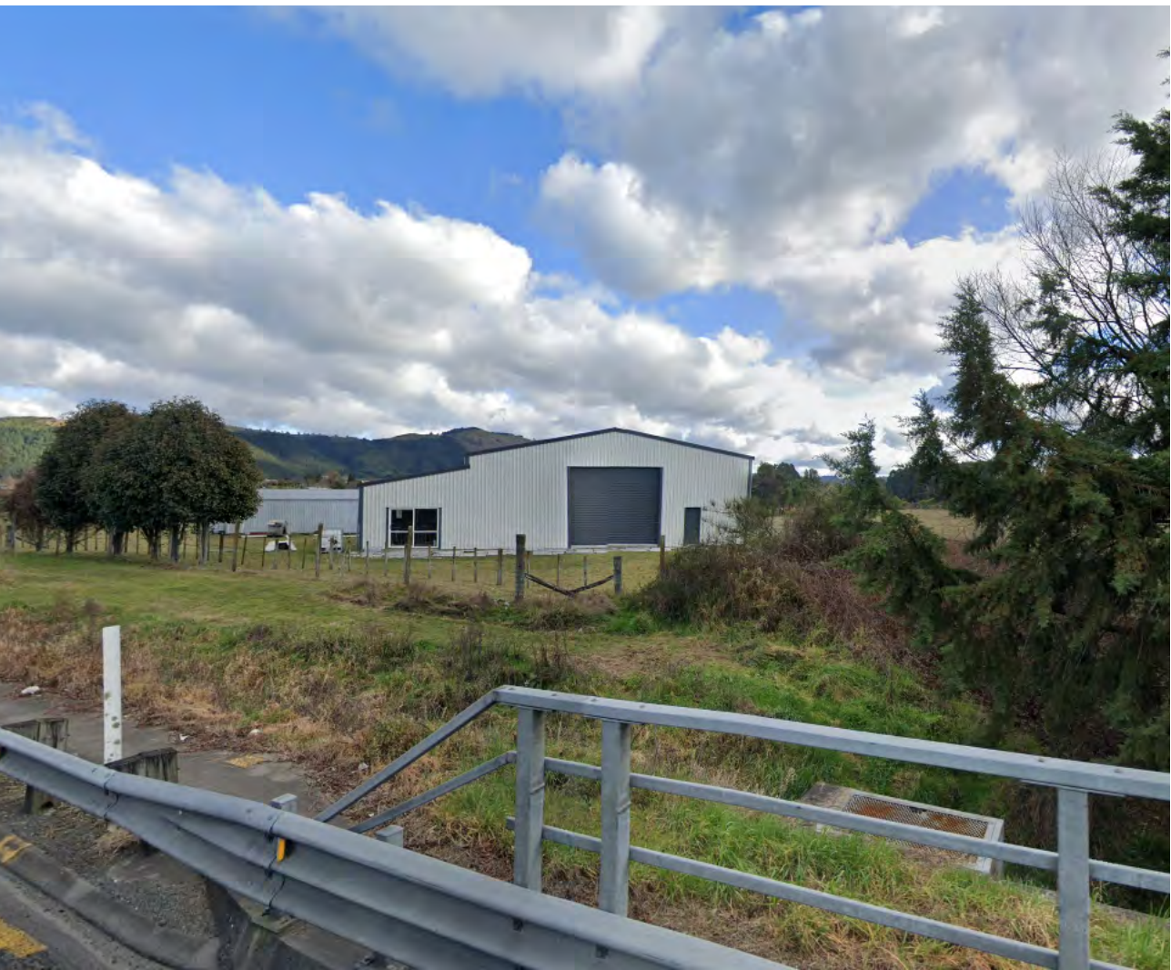
3 LOOKING SOUTH-WEST TOWARDS 31 NGONGOTAHA ROAD ON NGONGOTAHA ROAD.
