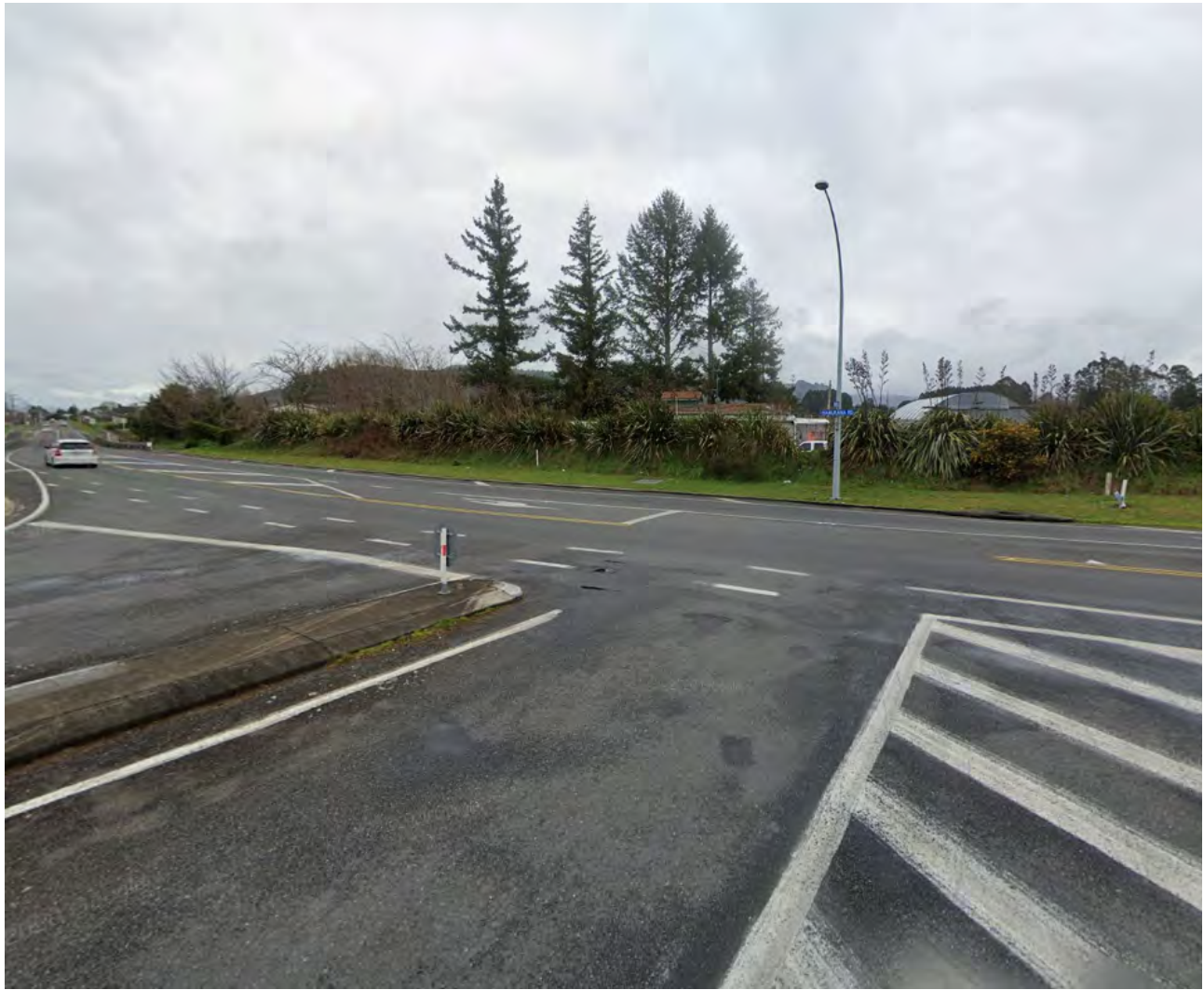
4 LOOKING SOUTH-WEST TOWARDS 31 NGONGOTAHA ROAD ON WAITETI ROAD.
