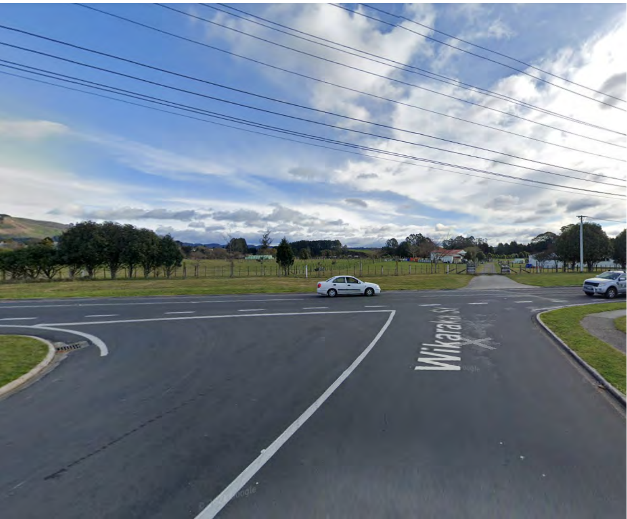
2 LOOKING WEST TOWARDS 31 NGONGOTAHA ROAD ON WIKARAKA STREET.
