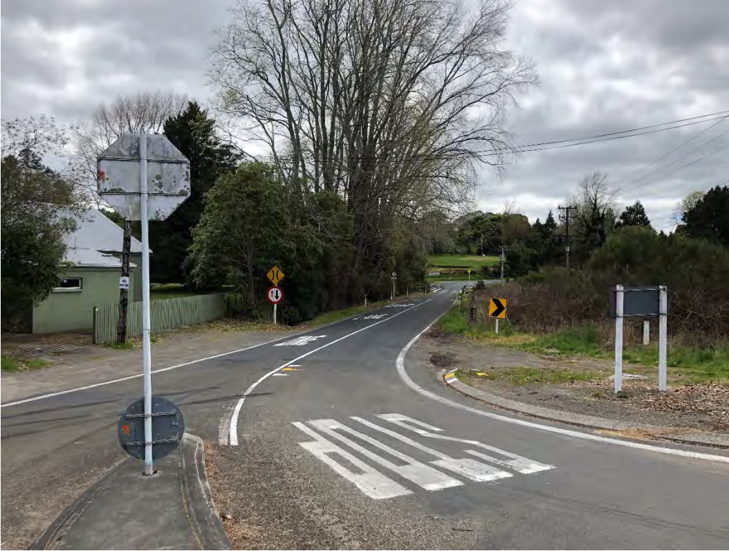
Photograph 2-11: Northbound approach to one-lane Bridge on Central Road
