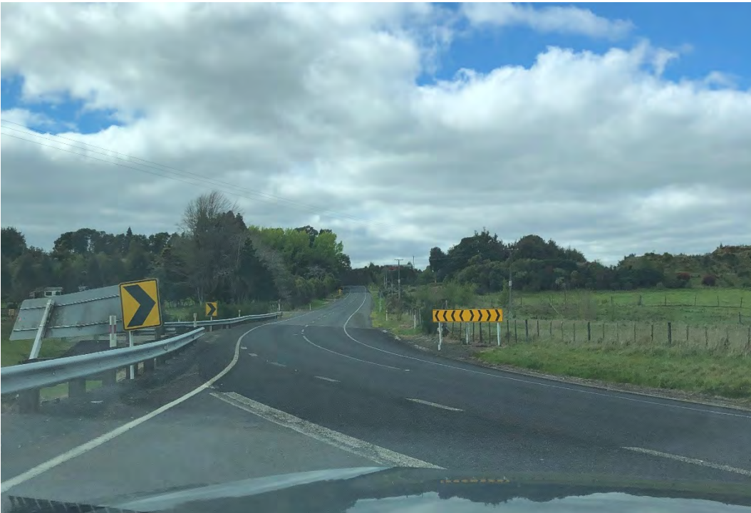
Photograph 2-9: SH36 / Jackson Road Intersection - Sightline North
