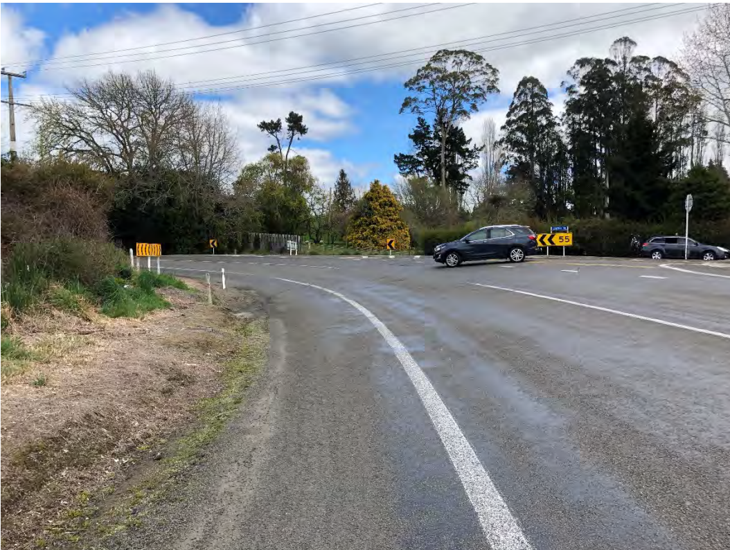
Photograph 2-13: SH36 / Central Road Intersection
