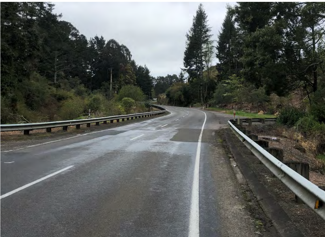
Photograph 2-4: SH36 View north
