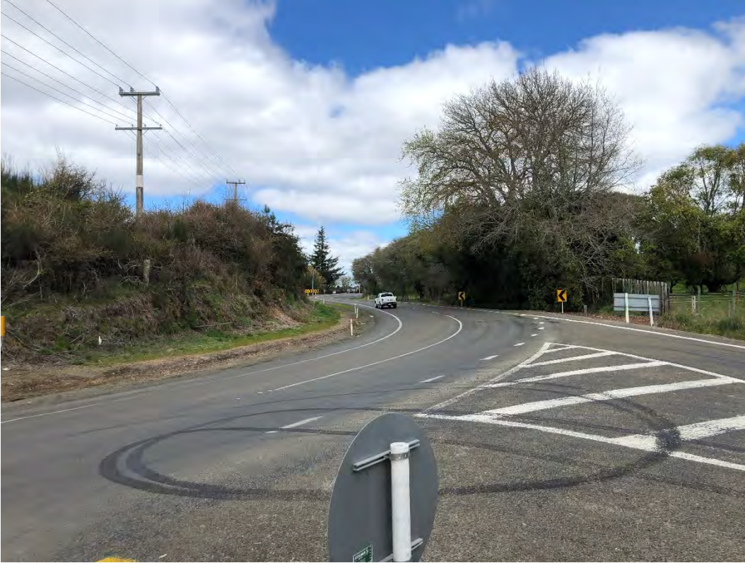
Photograph 2-12: SH36 / Central Road intersection
