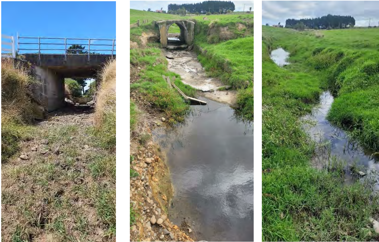
Figure 19: Watercourse 6 present on site is intermittent. It contains a large, perched concrete culvert approximately 3 m long with an additional 8 m of concrete lined channel in the watercourse bed. The watercourse is approximately 2 m wide at this point. There are a range of gravel and rock substrates in this watercourse outside of this area, with unstable banks subject to mass wasting.
