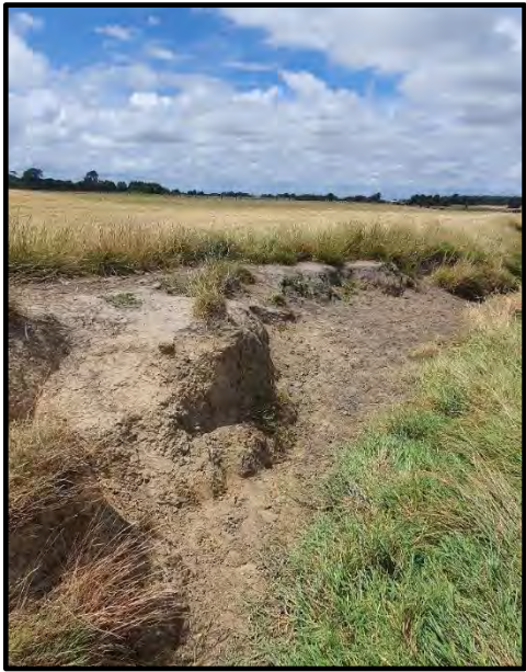
Figure 14: Example of over steepened slopes near watercourse resulting in small scale failures.
