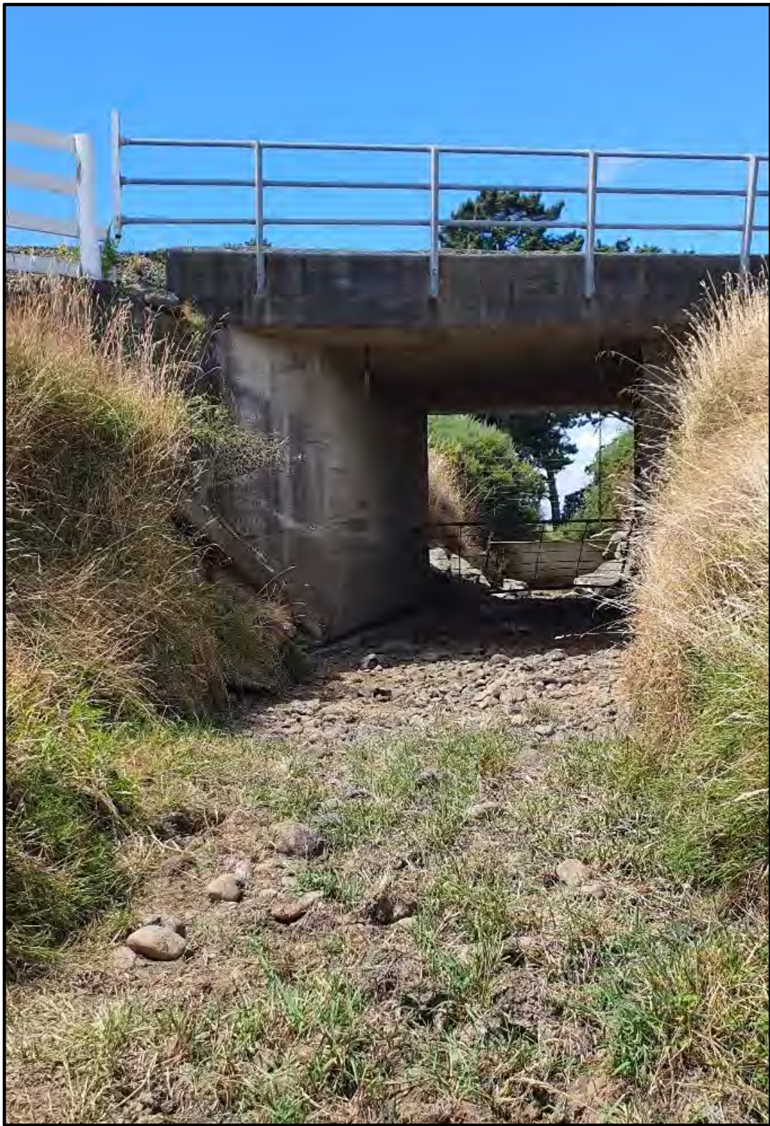
Figure 12: Site photograph showing the presence of cobbles in the near surface soils.
