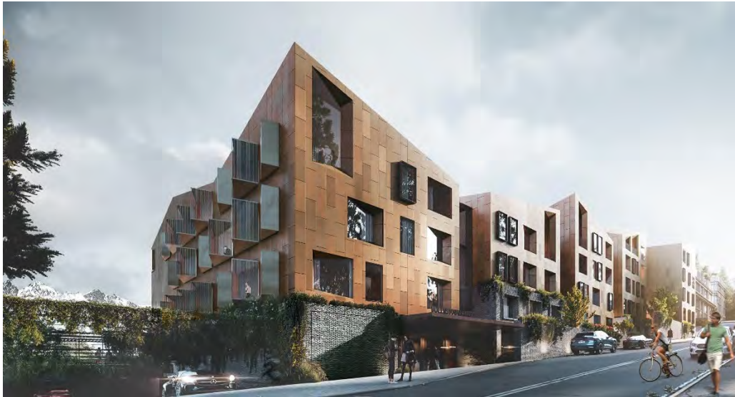
Figure 17 - Looking towards vehicle entrance from Man Street (by Woods Bagot)
