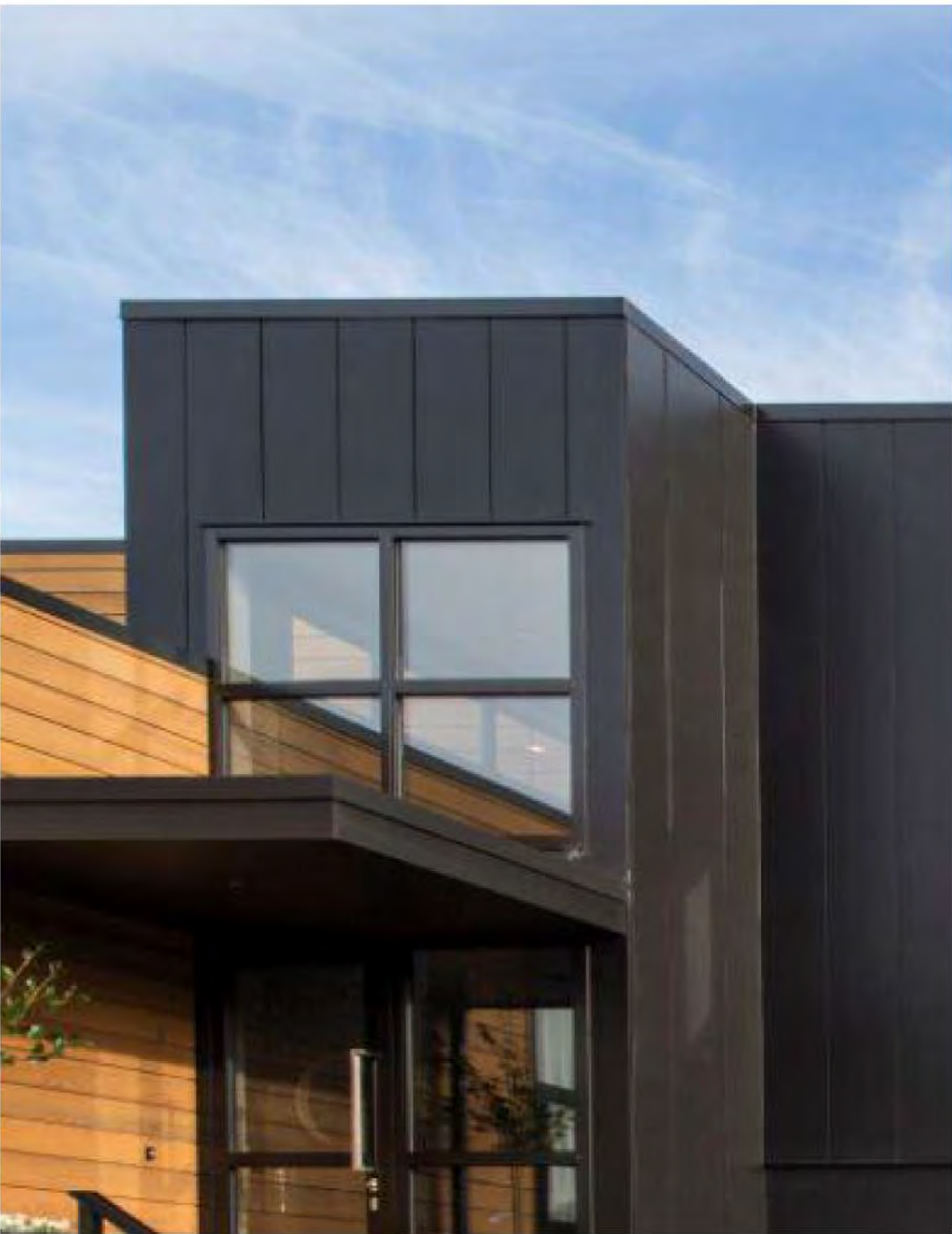
PAINTED FIBRE CEMENT SHEET
