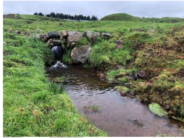
Photo L: A perched culvert within stream S4 likely resulting from channelisation of flows, these conditions can be problematic for fish passage
