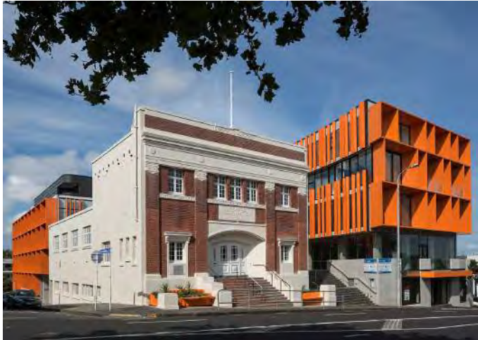
The Orange building on Newton Road
