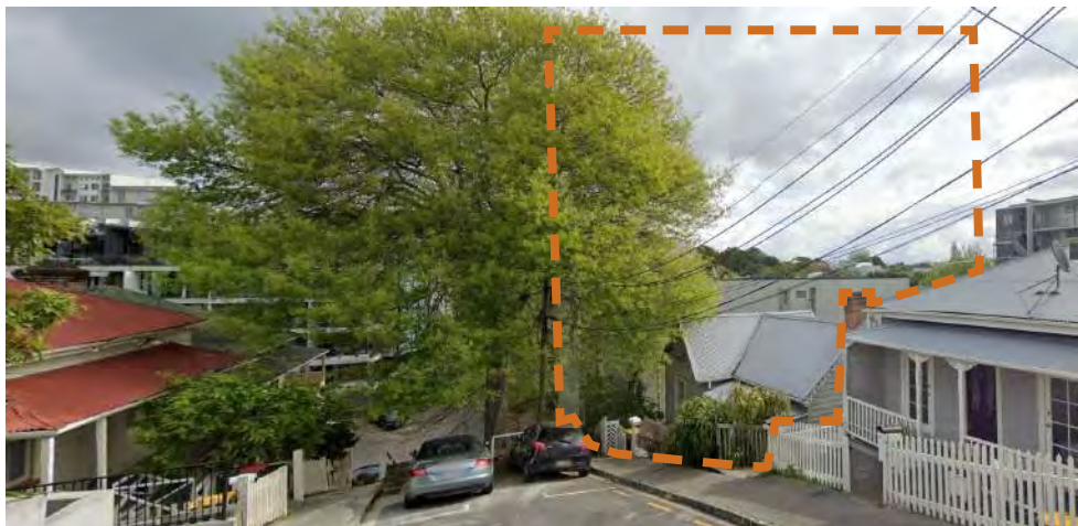
Site from Fleet Street North (Upper)
