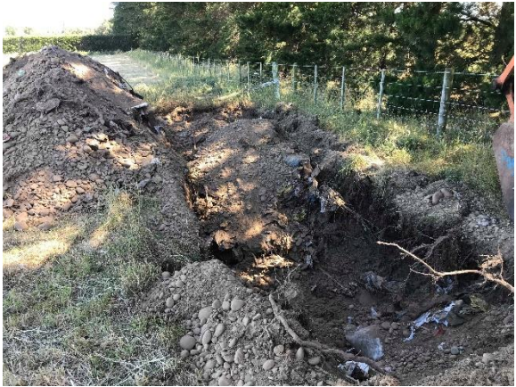
Photo 16: Extent of waste pit looking north
