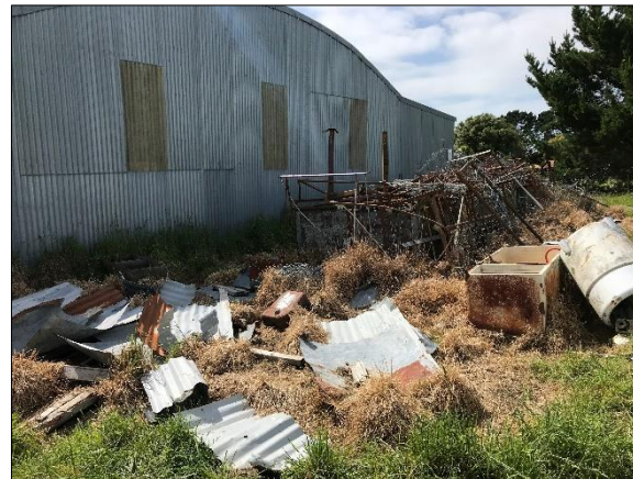
Photo 5: Storage of metal, wood and old appliances
