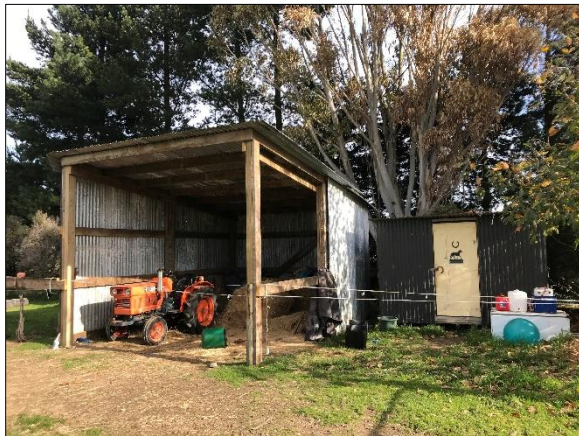
Photo 4: 4. Shed along south-western boundary line
