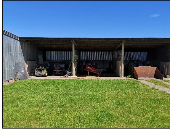
Photo 2: Shed on site
