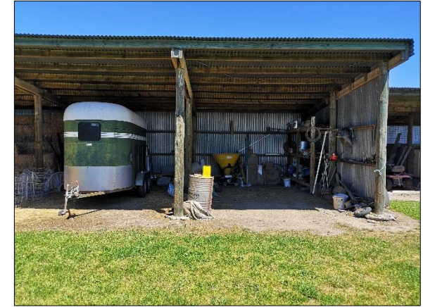
Photo 3: Shed on site
