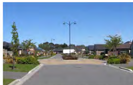
Traffic calming device which does not endanger cyclists and pedestrians
