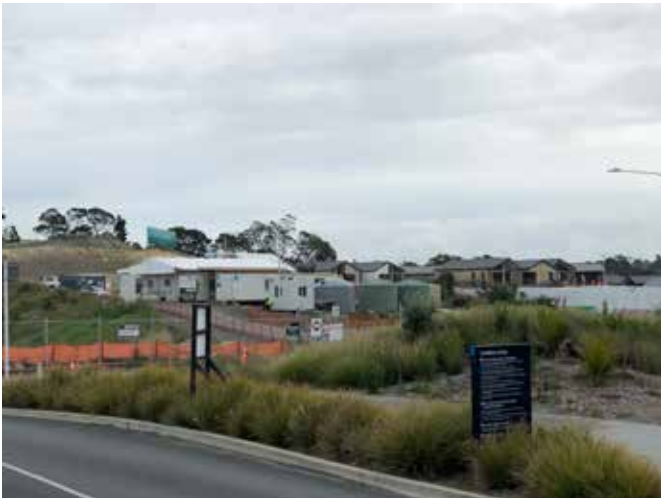
Above: The Botanic retirement village (west of the site) under construction.
