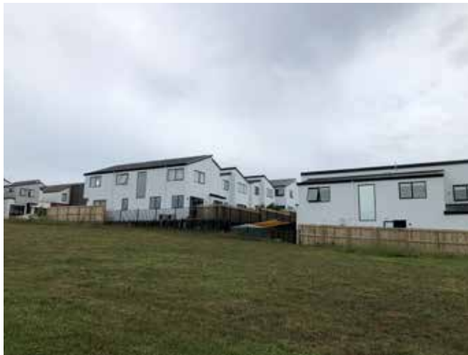
Above: Retaining wall transitions in Stage 1 aligned at rear garden boundary.
