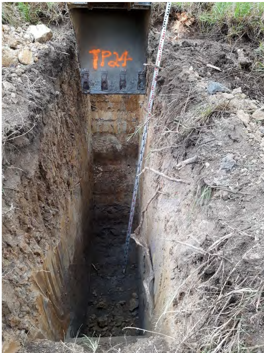
TP24-20 – TEST PIT EXCAVATION
