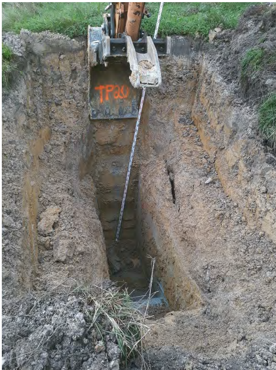
TP20-20 – TEST PIT EXCAVATION
