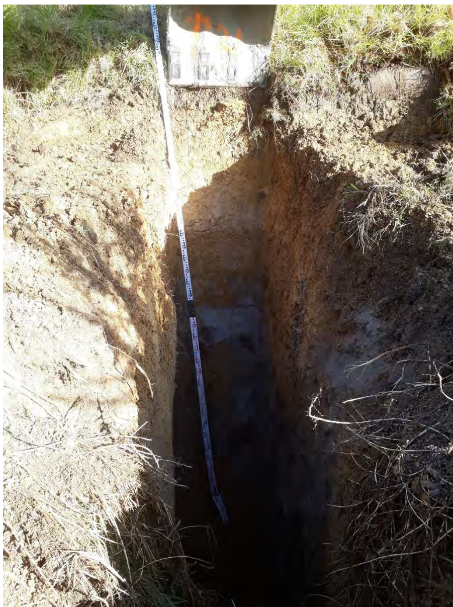
TP21-20– TEST PIT EXCAVATION
