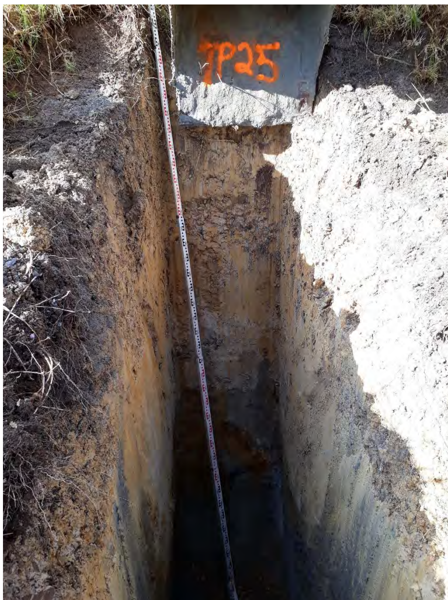
TP25-20 – TEST PIT EXCAVATION
