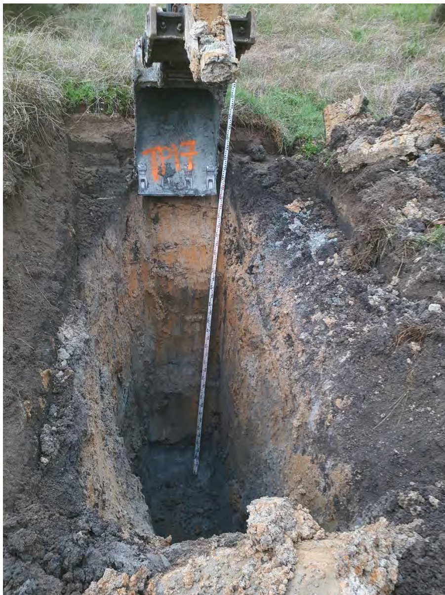
TP17-20 – TEST PIT EXCAVATION
