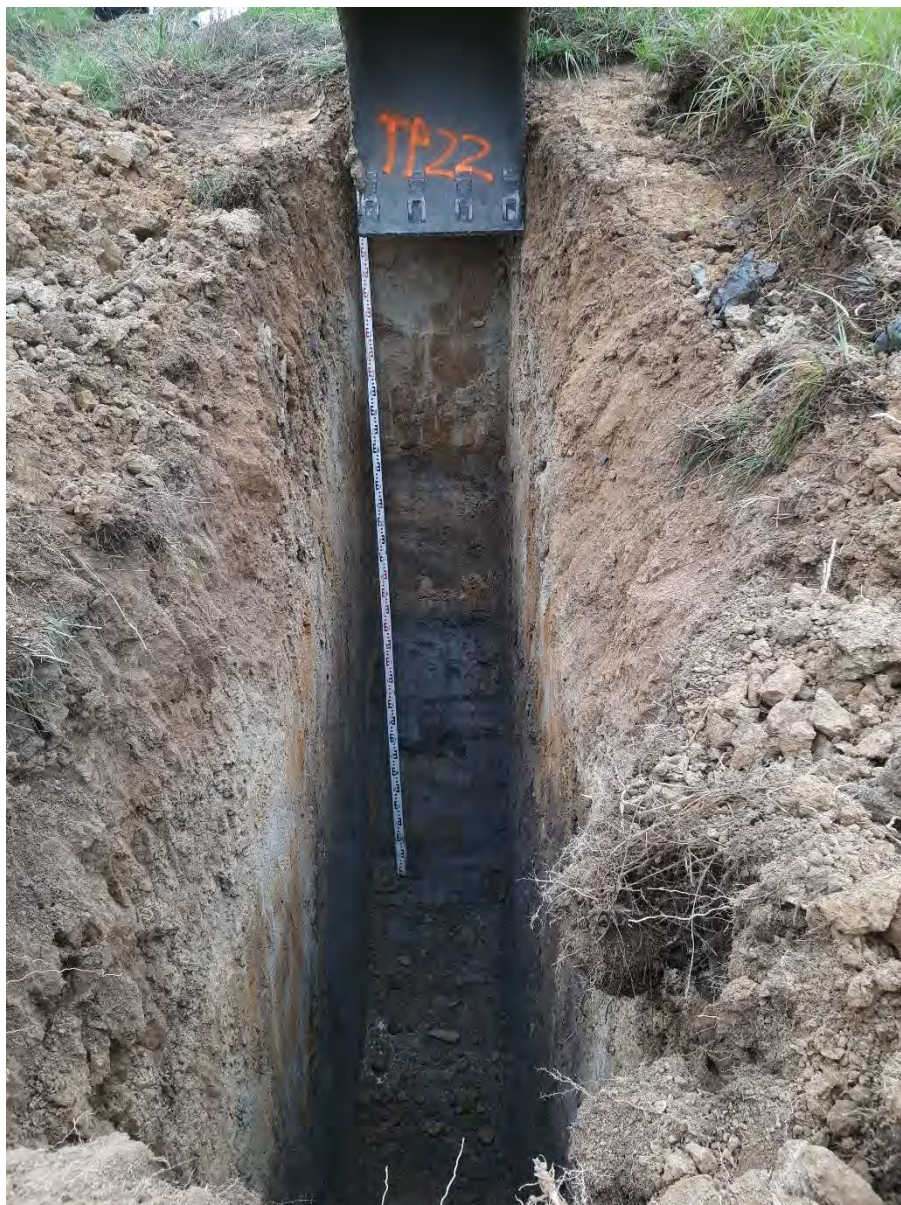
TP22-20 – TEST PIT EXCAVATION
