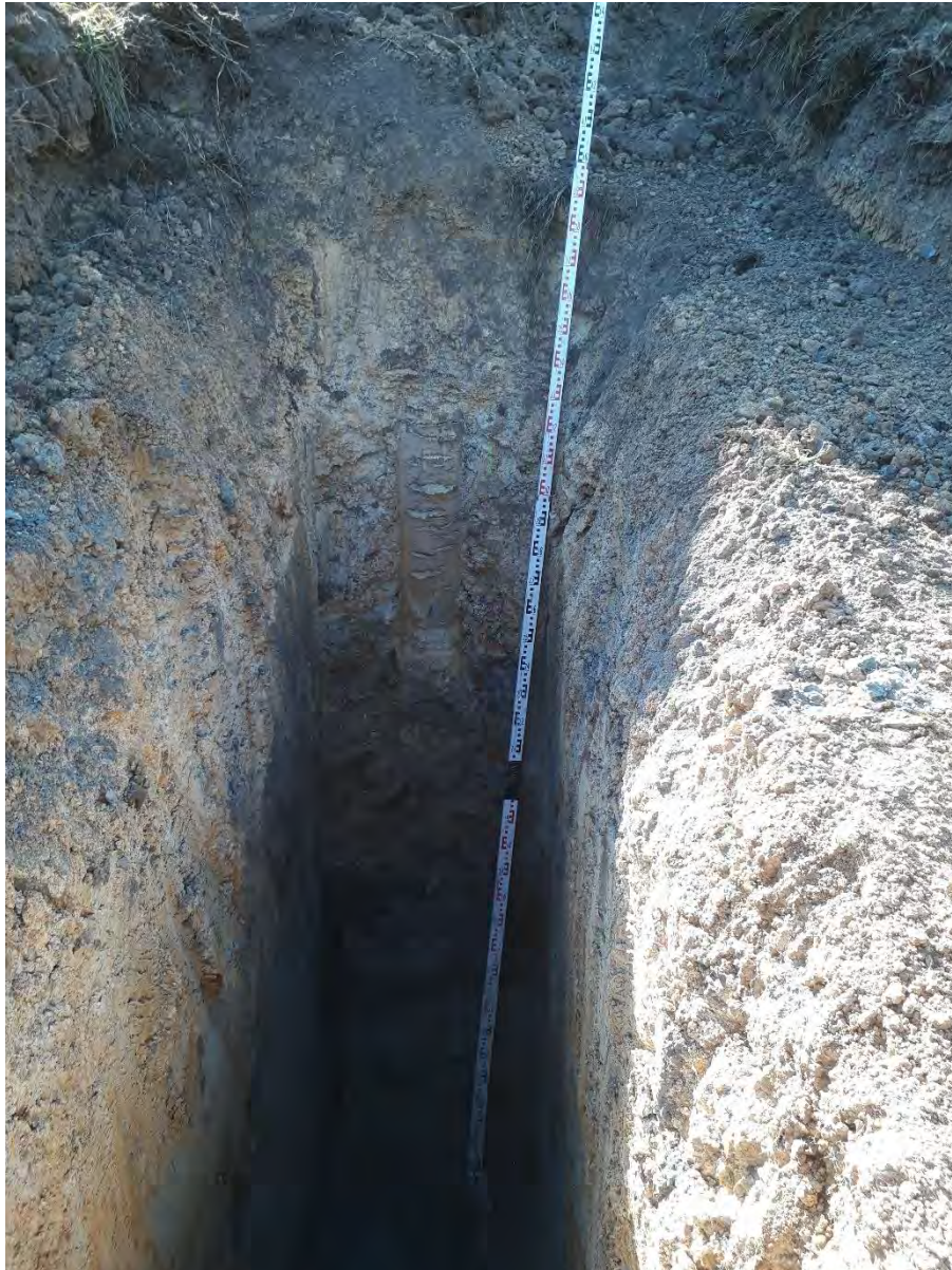
TP16 -20 – TEST PIT EXCAVATION
