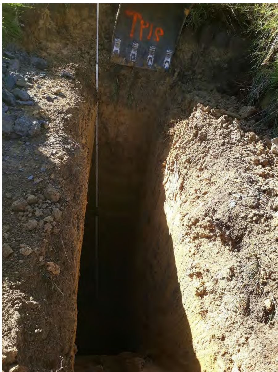
TP18-20 – TEST PIT EXCAVATION
