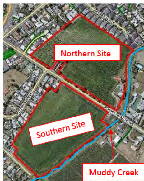
Figure 1: 2022 Aerial Site Photo (Source: Hastings District Council (HDC) GIS)
