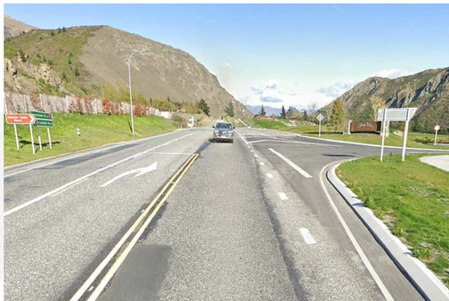
Photograph 3: Gibbston Highway / Vines Way Intersection (Looking West)
