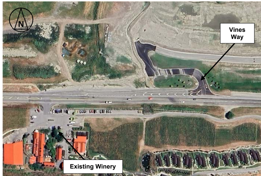
Figure 3: Aerial Photograph of Entry into Gibbston Winery / Restaurant and Vines Way Intersection Serving the Site
