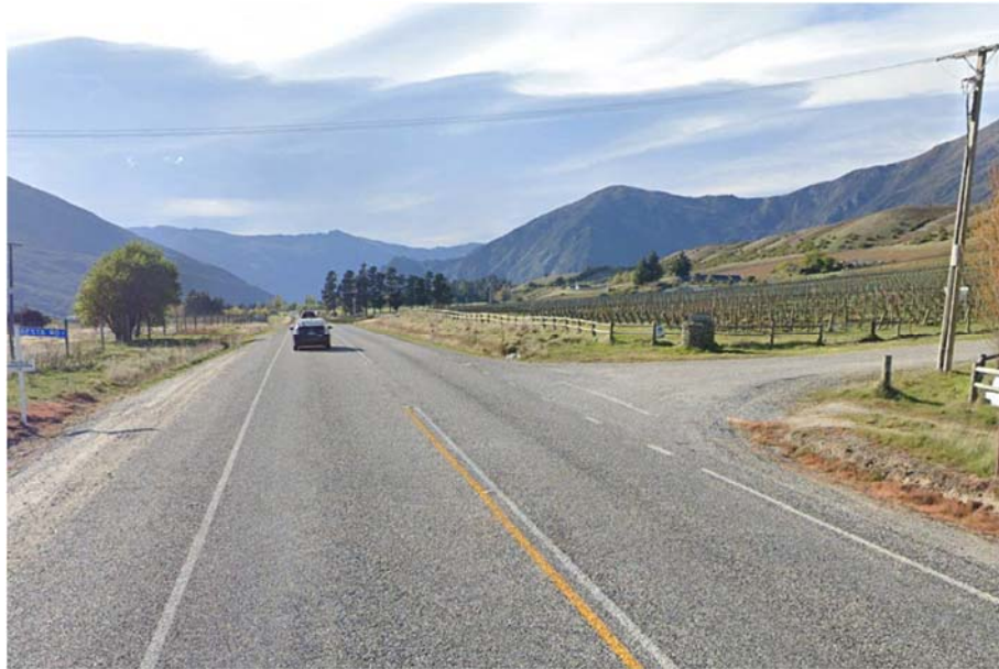
Photograph 4: Existing Access Intersection into Northern Side of the Site (Looking West)
