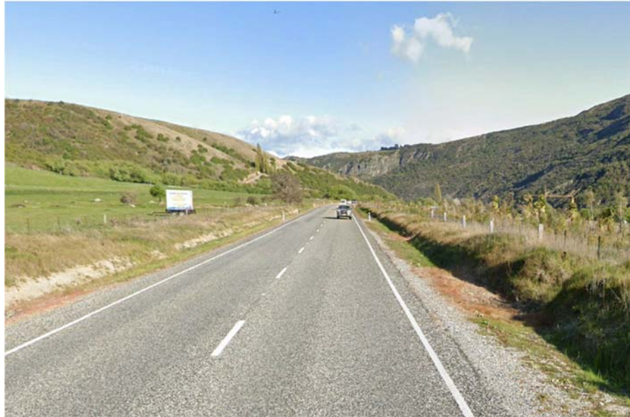
Photograph 1: Typical Cross Section of Gibbston Highway Looking East
