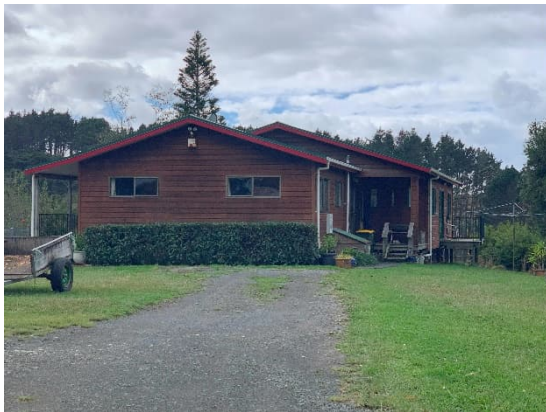
Photograph 3. View of main dwelling at 55 Russell Road, stained wooden weatherboard cladding
