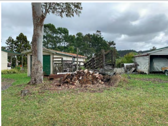
Photograph 5. Example of sheds between dwellings at 55 Russell Road, single garage to left is clad with suspected ACM.
