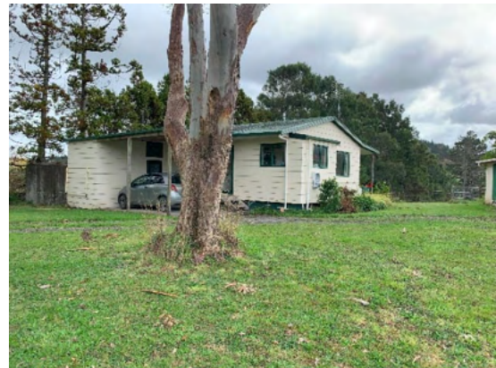
Photograph 4. View of minor dwelling at 55 Russell Road, modern fibre cement cladding.
