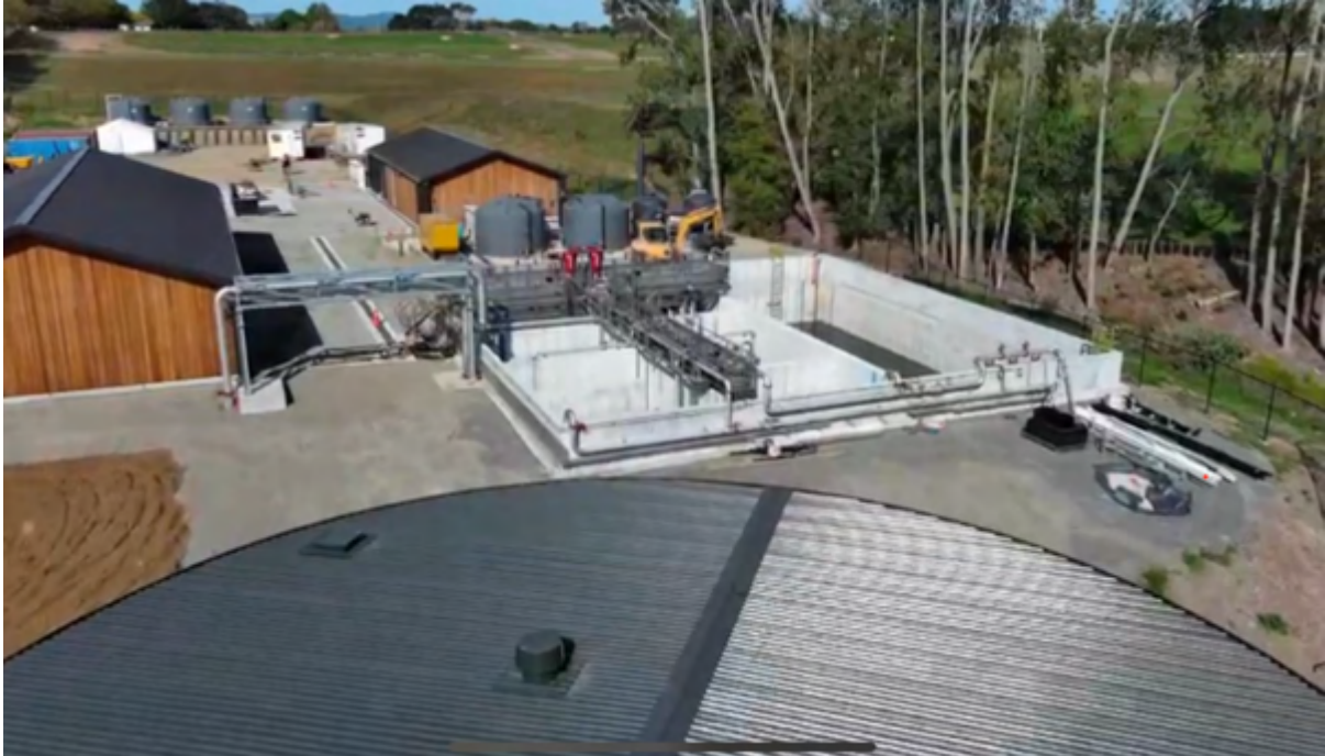
Figure 5 Apex Water 1,200-house subdivision MBR wastewater treatment plant featuring acoustically isolated plant room with full odour extraction and treatment.
