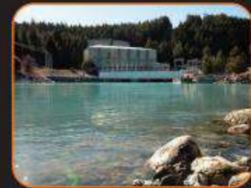
TEKAPO A POWER STATION One 25 MW Unit. Commissioned 1951
