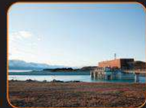
TEKAPO B POWER STATION Two 80 MW Units. Commissioned 1977
