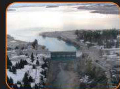
LAKE TEKAPO CONTROL STRUCTURE (Gate 16)
