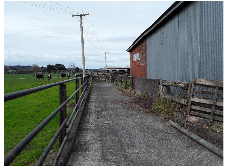
Corrugated Metal Shed (1) - Eastern Side
