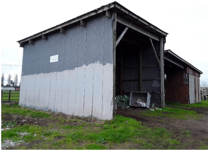
Corrugated Metal Shed (1)
