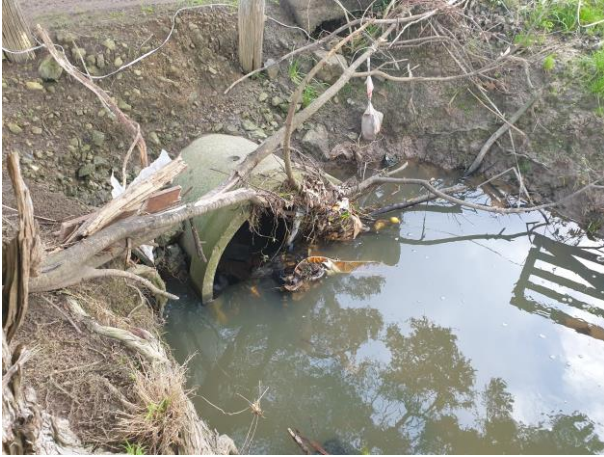
Photo 12. An embedded culvert is present within the stream channel
