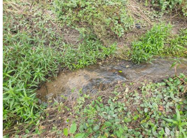
Photo 37. Some sections of the stream bank contained connectivity to the floodplain.
