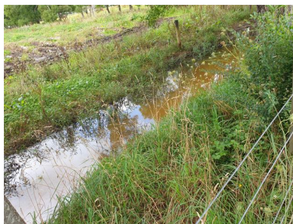
Photo 61. The downstream reach contained standing water.
