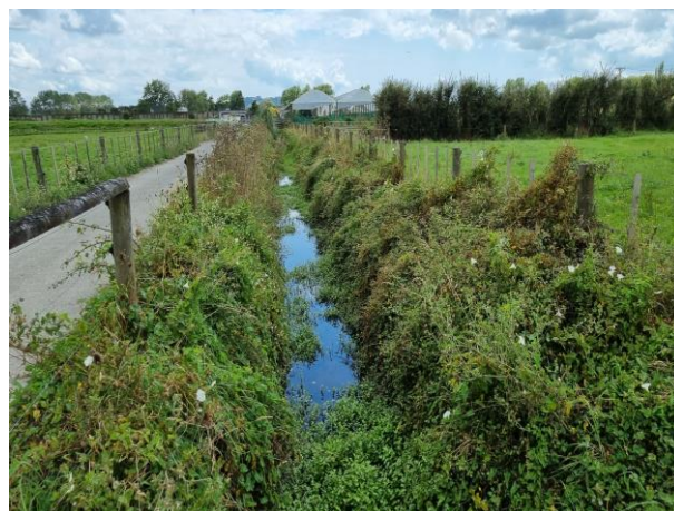
Photo 27. Downstream reach of Watercourse 2
