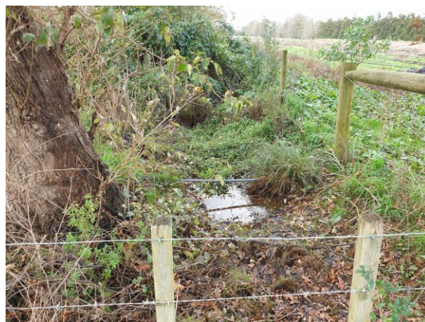
Photo 41. Drain k (northern reach)
