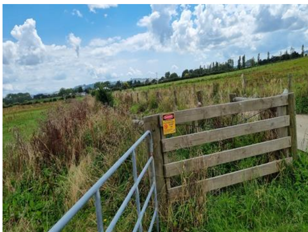
Photo 42. Drain k (eastern reach)
