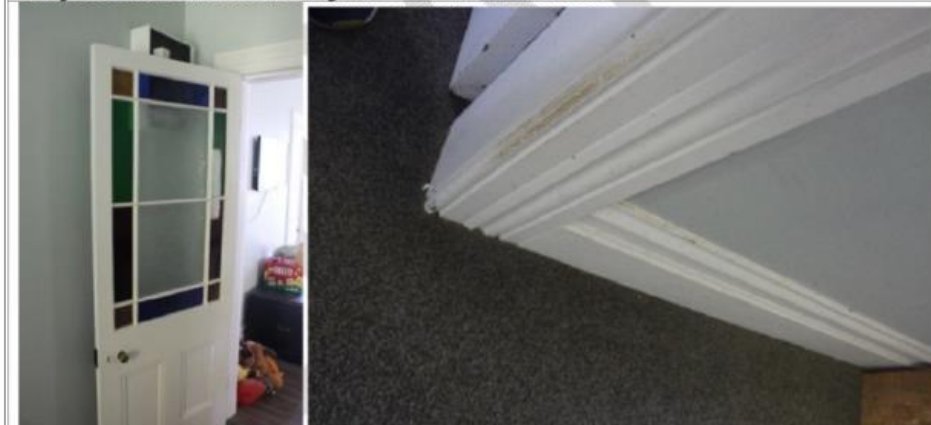
Interior joinery details
