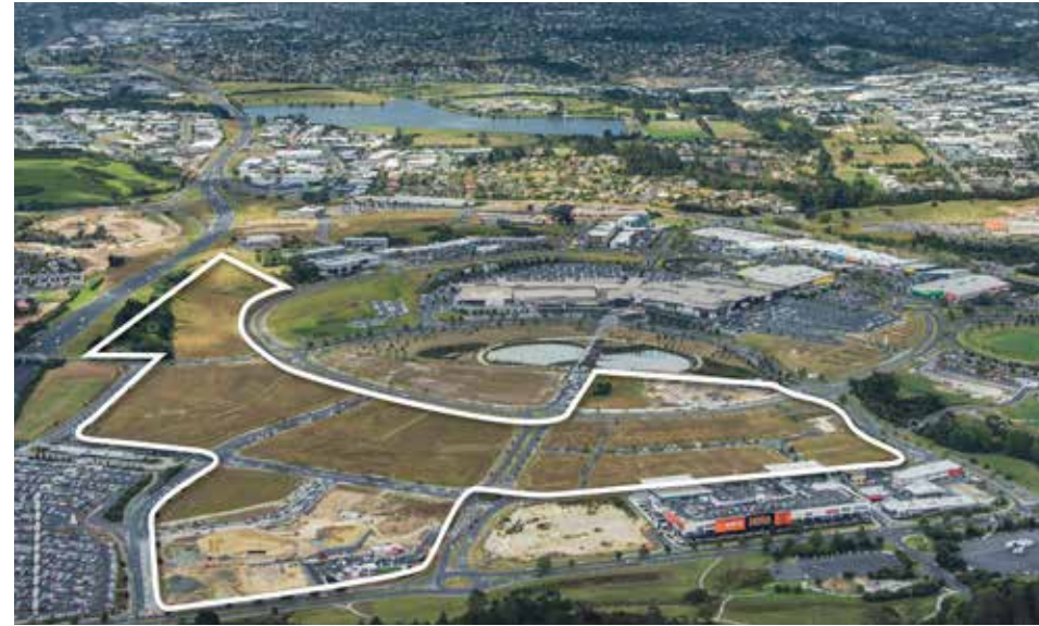
A large scale mixed use land subdivision located at Albany Town Centre, Albany, New Zealand.
