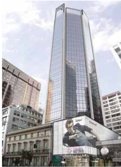
A 27 level 'A' grade office tower located at 125 Queen Street, Auckland CBD, New Zealand.
