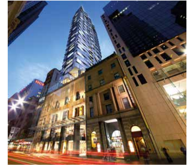
A 38 level, 200 unit residential apartments, 4,500m 2 commercial and 3,200m 2 retail development located in York & George, Sydney CBD, Australia.
