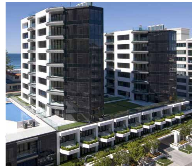
Eleven Apartments, a 65 unit apartment development located in Mt Maunganui, New Zealand.
