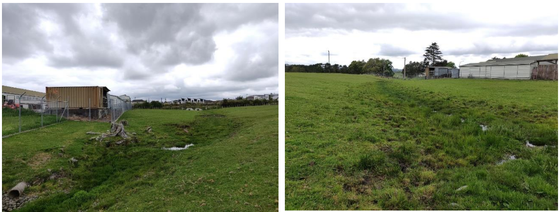
Figure 15. South-eastern creek on 102-102A Totara Road, looking along eastern property boundary and facing south towards the boundary showing concrete culverts (left); and south-eastern creek on 102-102A Totara Road, facing north/northeast with eastern property boundary on right (right)
