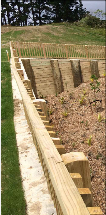
WALL FENCING EXAMPLE (WOODEN 50% VISUALLY PERVIOUS)
