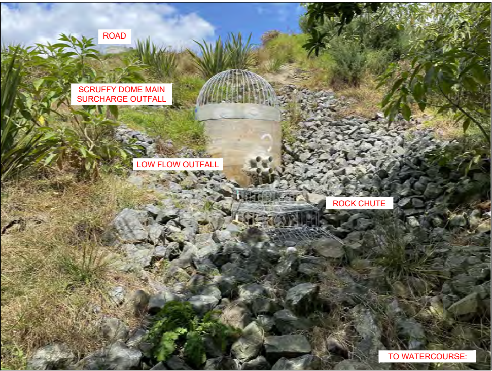
EXAMPLE BUBBLE UP OUTFALL AND ROCK CHUTE.
