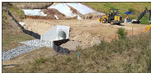
OPTION 1 - PIPE CULVERT
