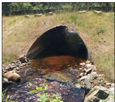
OPTION 3 - PIPE-ARCH CULVERT
