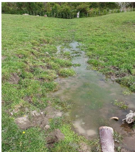
Photo 14. Stormwater pipe and stagnant puddle at the top of Watercourse C.2
