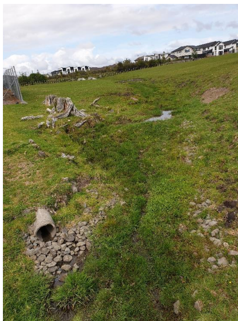
Photo 4. Upstream view of Watercourse A with a stormwater pipe present
