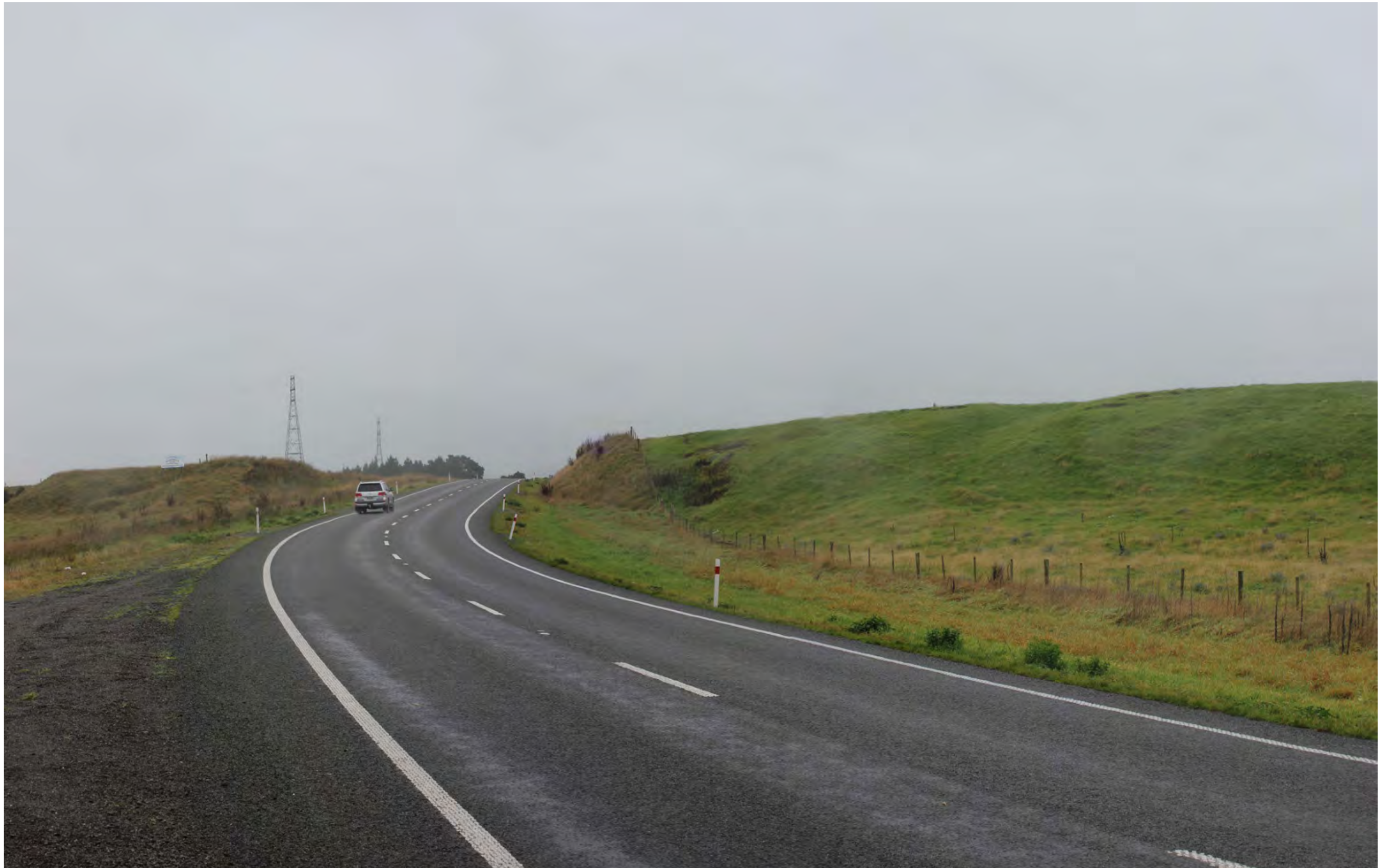
Photo 12: View north east from Waipara Flat Road
